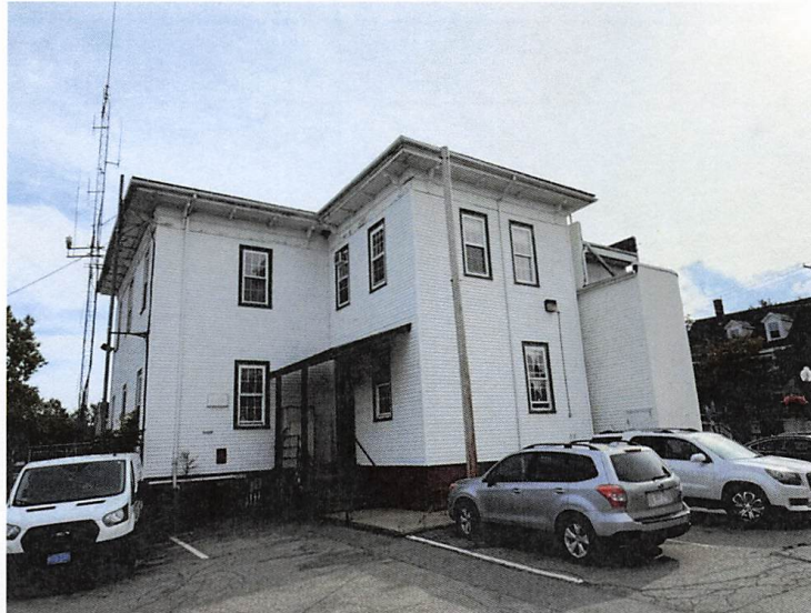
Looking southwest at 1884 addition
