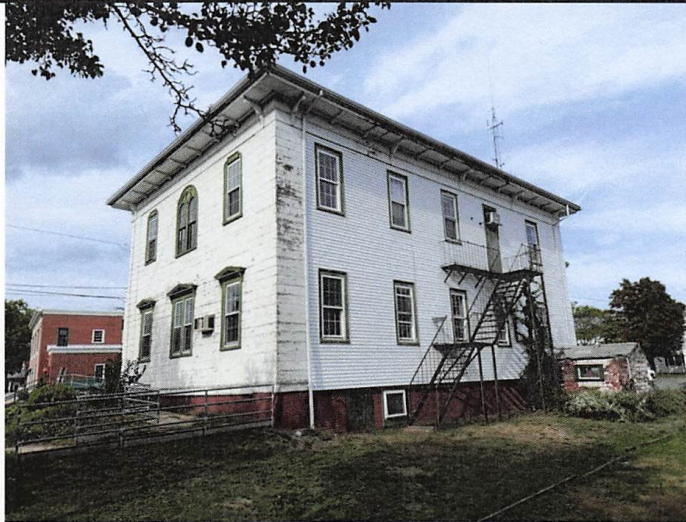
West (façade) and south elevations
