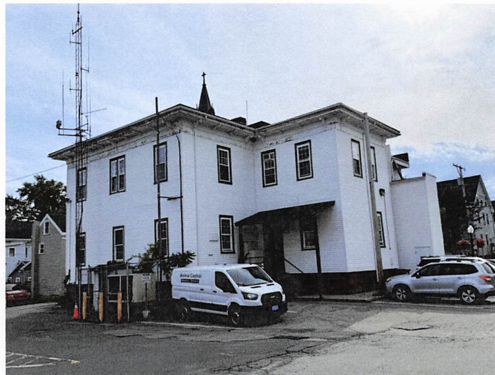
Looking SW at rear (east) and north sides
