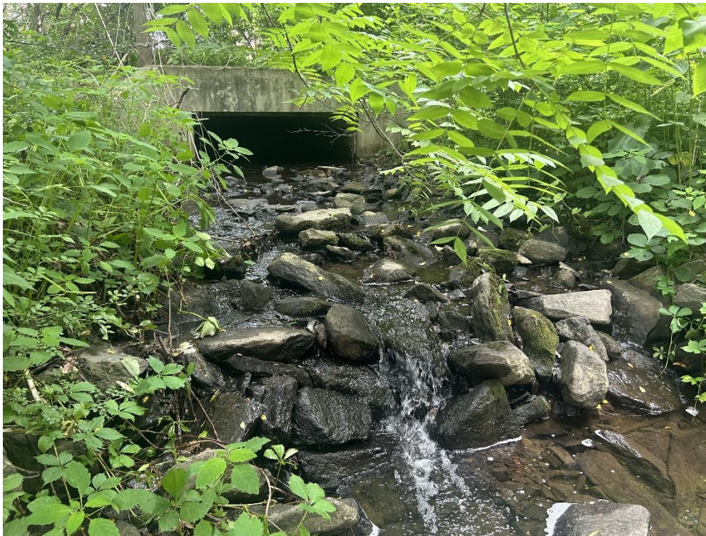
Photograph No. 4: A northerly view of the outlet of the subsurface stream (Wetland B) on Site.
