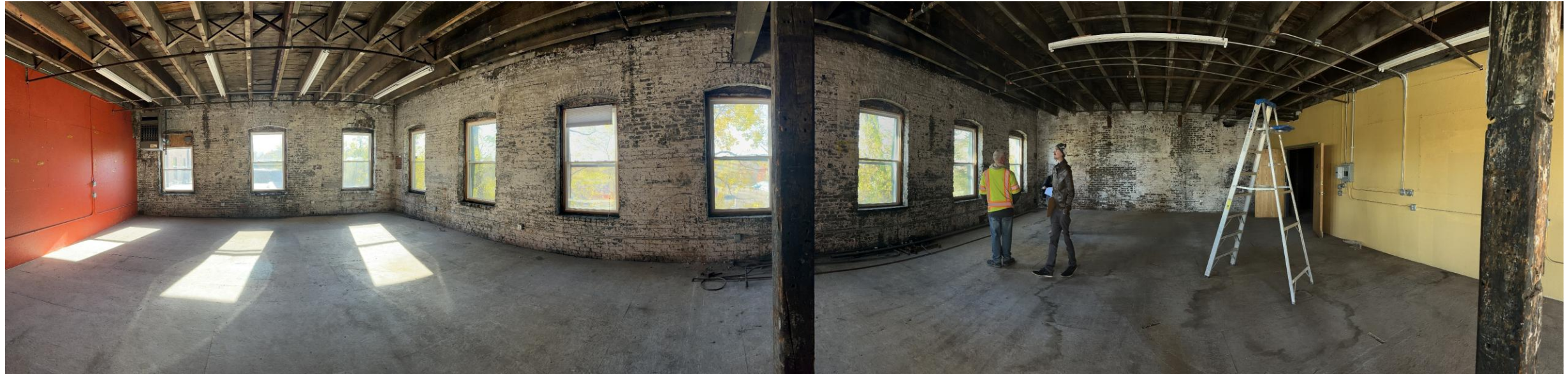
Existing Conditions- Interior
