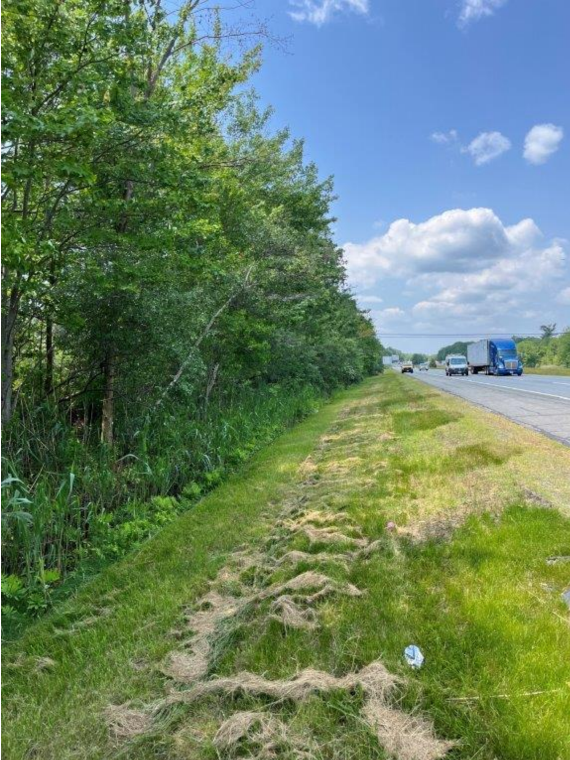
Photo 7: View facing west of the excavated drainage ditch following reestablishment of vegetation in July 2025.
