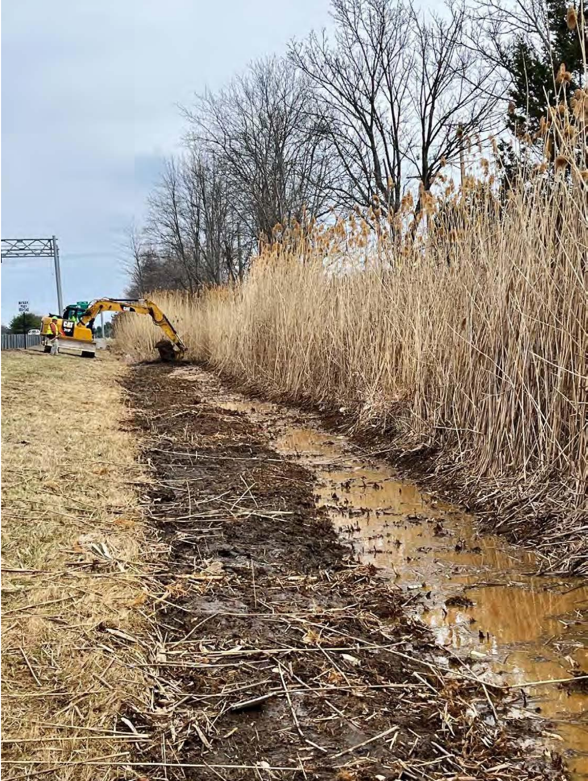
Photo 2: View facing east of the excavated drainage ditch during excavation in April 2025. This location is approximately adjacent to the driveway access point to 14 South Hunt Road.
