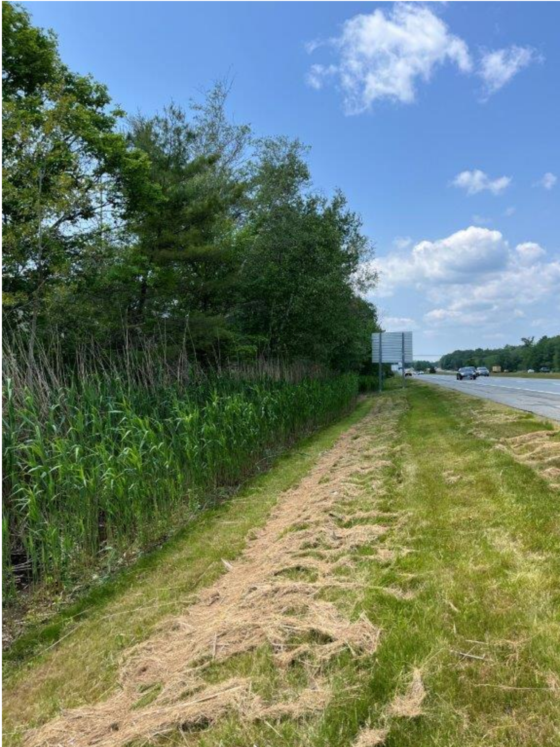
Photo 4: View facing west of the excavated drainage ditch following reestablishment of vegetation in July 2025.
