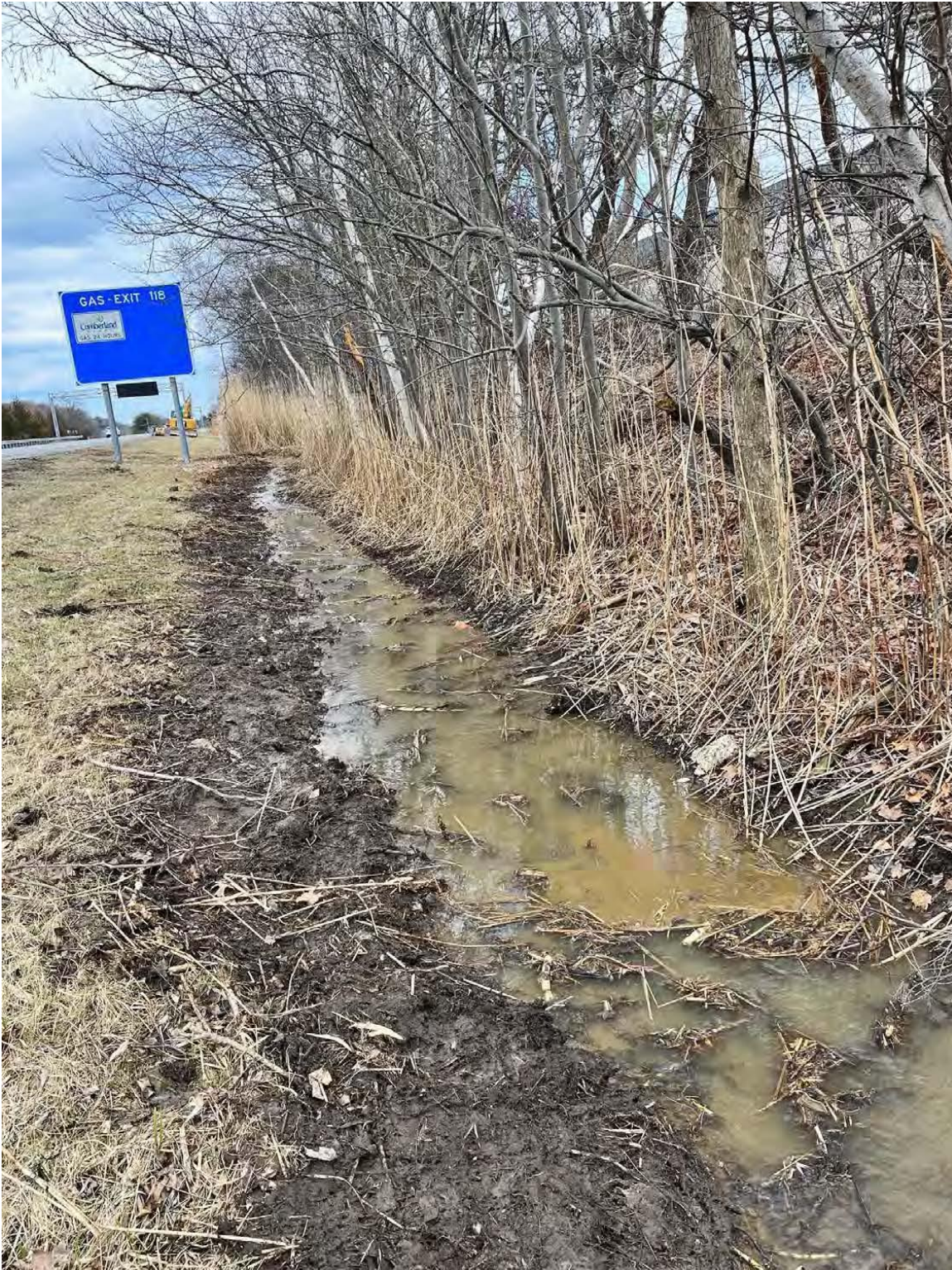
Photo 1: View facing east of the excavated drainage ditch during excavation in April 2025. This location is approximately adjacent to 16 & 18 South Hunt Road.
