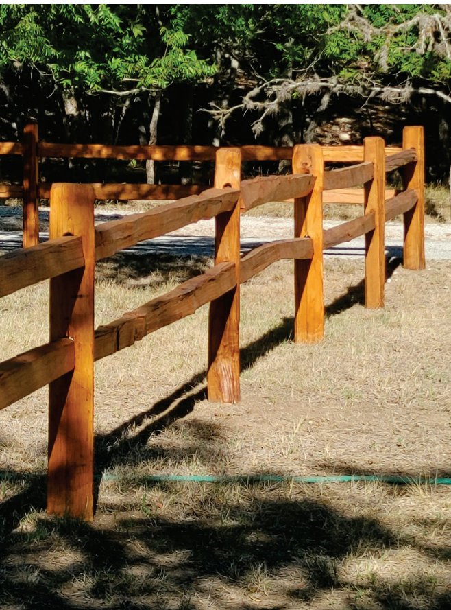
Split Rail Fence Along Boat Ramp Property Line
