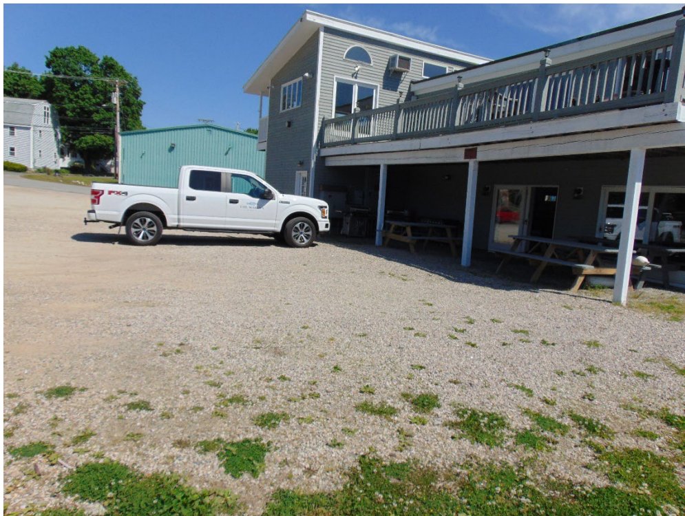
Photo 12 – View northerly from the retaining wall along the Merrimack River of the existing marina building and ground level access. The existing paved site driveway at Merrimac Street is located in the upper left of the photo.
