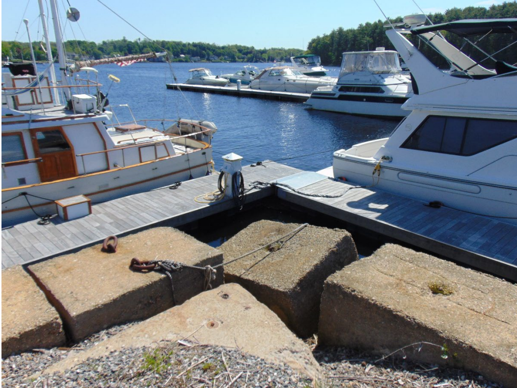
Photo 9 – View westerly of the existing retaining wall condition at the southeasterly corner of the site at the juncture of the Merrimack and Pow Wow Rivers.
