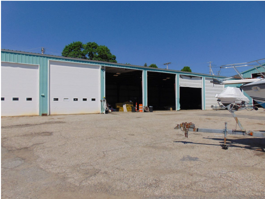
Photo 14 – View northwesterly of the existing westerly maintenance building to be removed and the ground level access.
