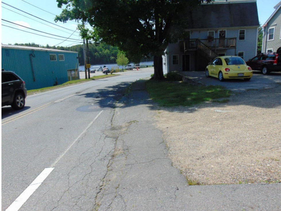
Photo 5 – View from the westerly side of Merrimack Street southerly of the existing gravel driveway to 13 Merrimac Street (Lot 82) and the existing 4-foot wide sidewalk and proposed 5-foot wide sidewalk reconstruction. The existing dwelling on Lot 82 can be seen in the upper portion of the photo.
