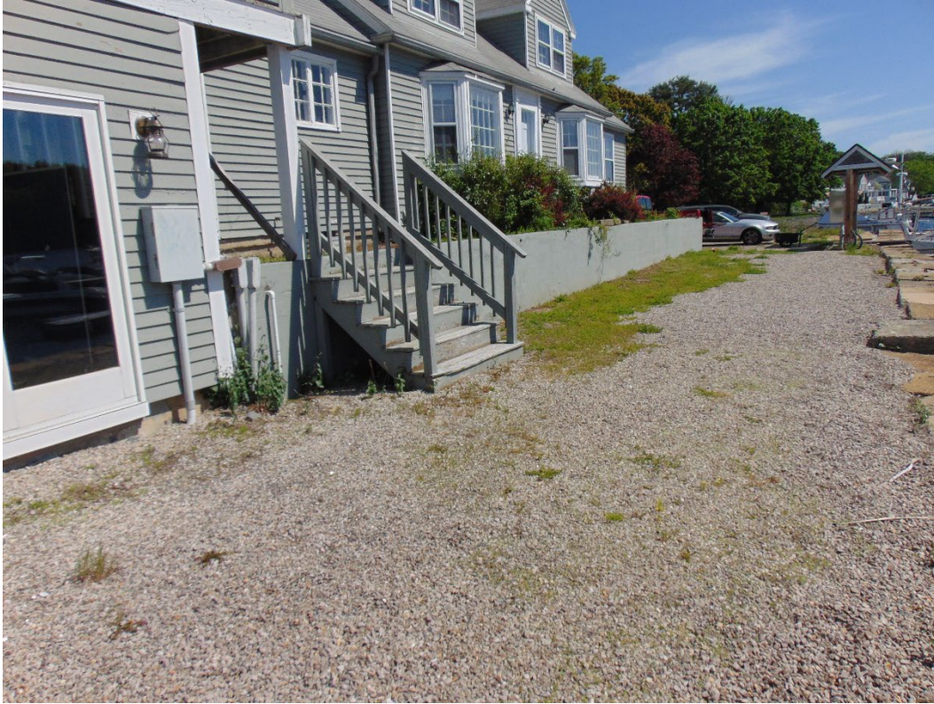
Photo 13 – View northeasterly from near the Merrimack River retaining wall of the ground level marina building access and the adjacent building with a retaining wall and stair access.
