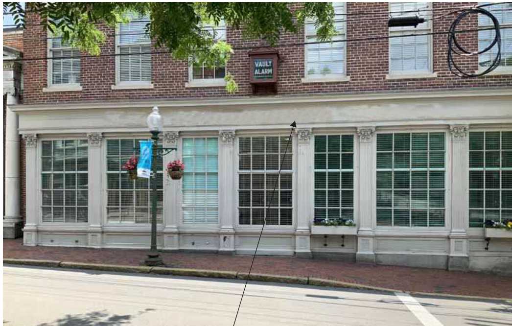
FILL EXISTING HOLES, NO SIGN REPLACEMENT
