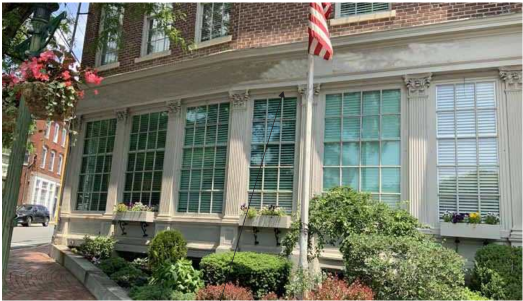
FILL EXISTING HOLES, NO SIGN REPLACEMENT
