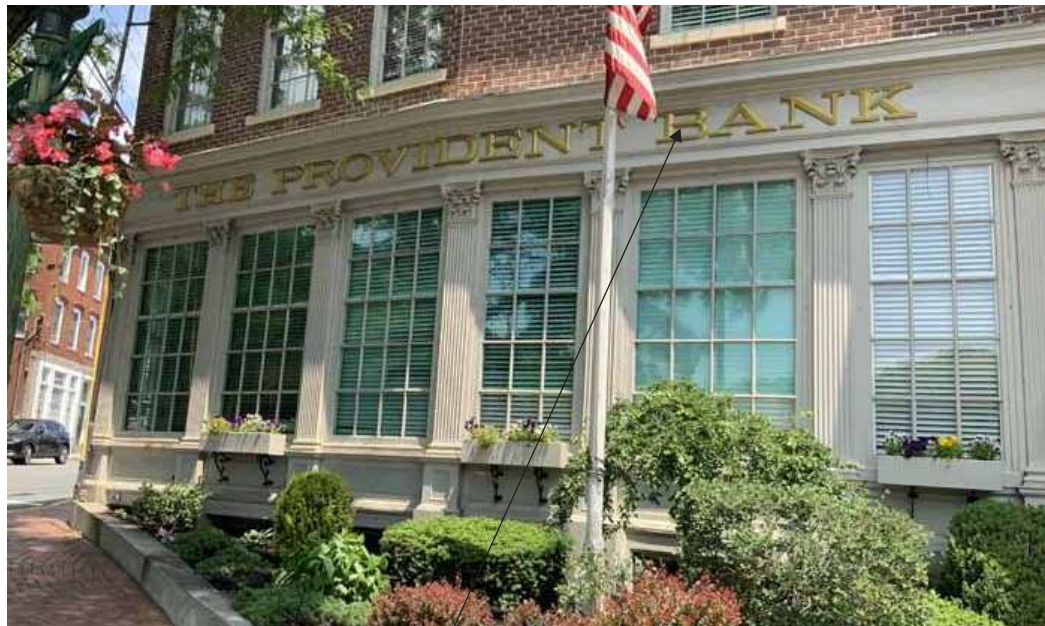
EXISTING SIGN TO BE REMOVED
