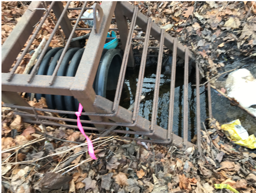
Photo 6: Upstream end of Friend Street Culvert.
