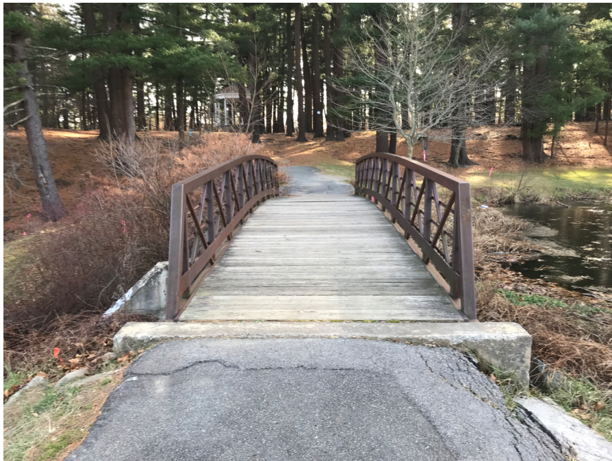
Photo 4: Footbridge over upper dam spillway.
