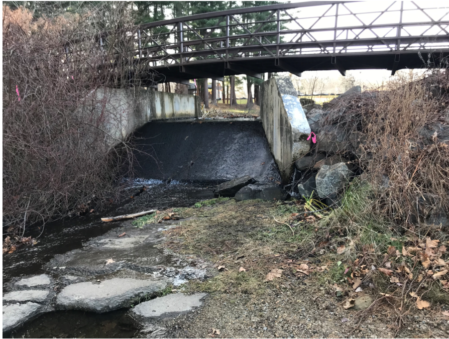
Photo 3: Downstream side of upper dam at Pleasure Pond.
