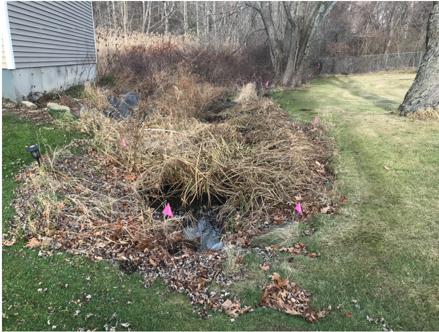
Photo 7: Upstream end of Lindbergh Avenue culvert.
