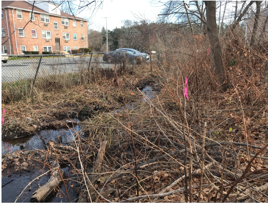
Photo 5: intermittent stream channel upstream of Friend Street culvert.
