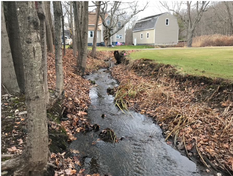
Photo 8: Channel downstream of Lindbergh Avenue culvert, facing upstream towards driveway.
