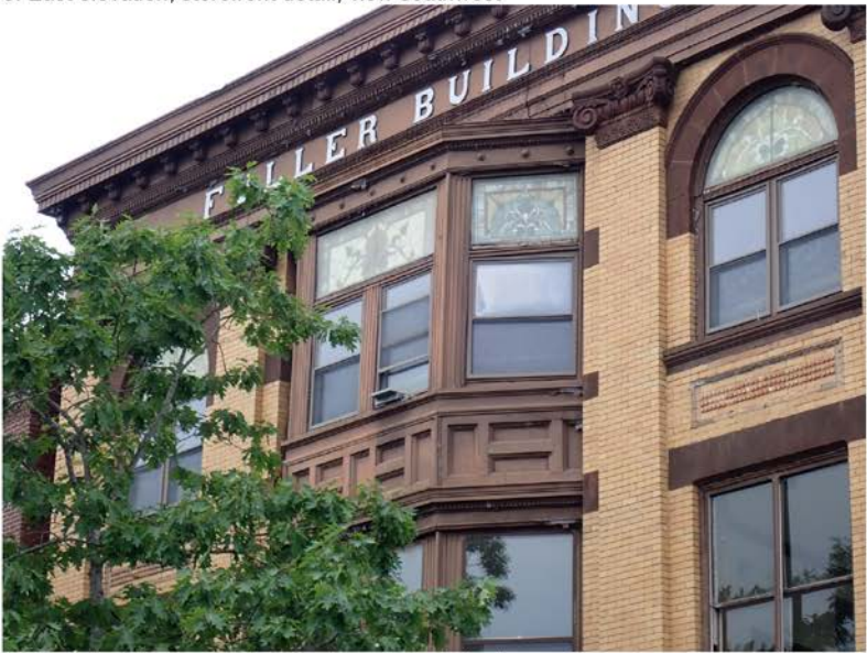
4. East elevation, upper floor and cornice detail, view southwest
