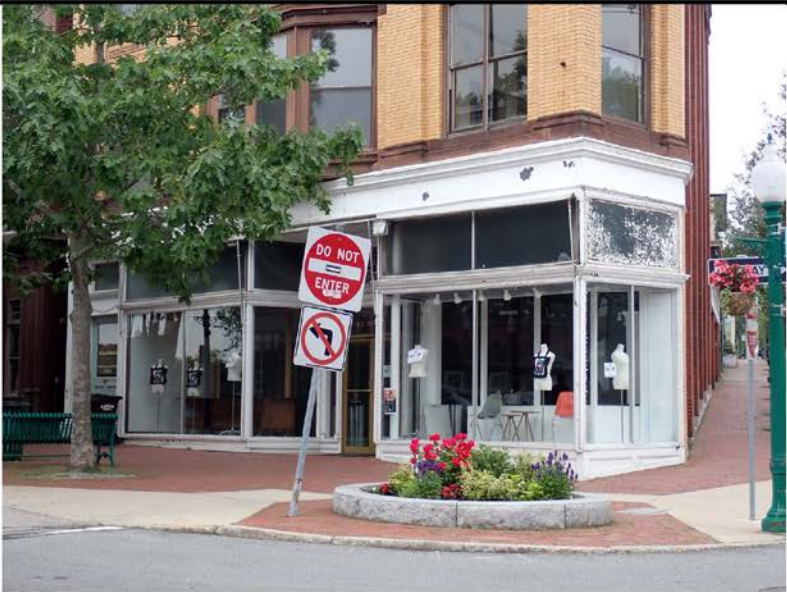
3. East elevation, storefront detail, view southwest
