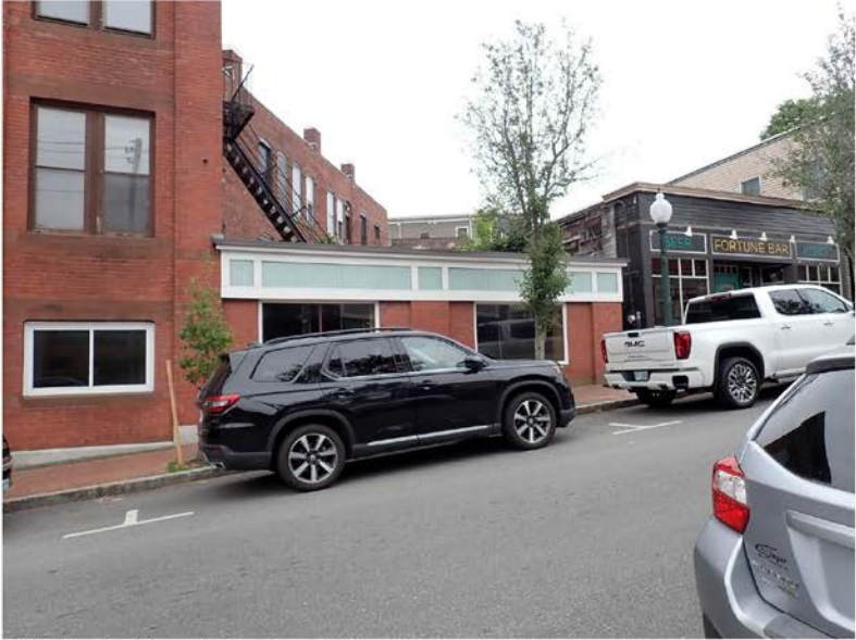
6. North elevation, single-story addition, view south
