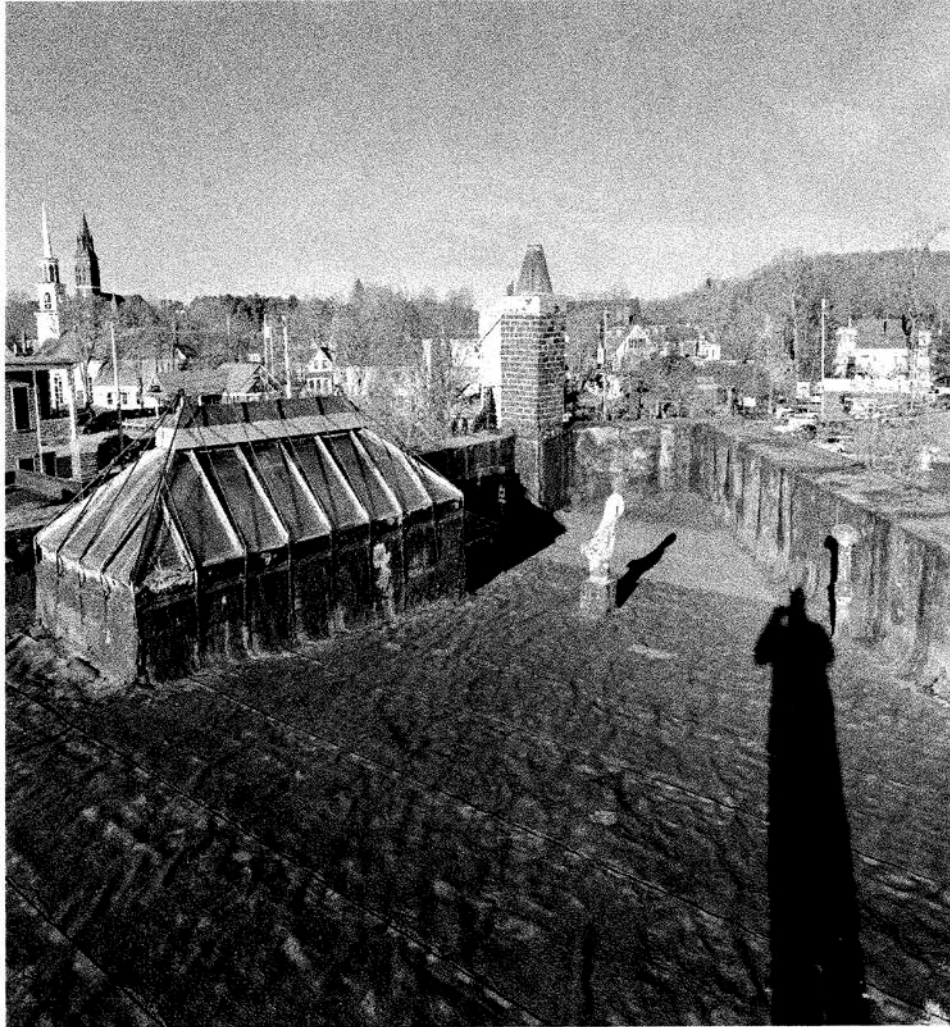
16. Roof Membrane Replacement – The roof membrane on the 1-story and 3-story building will be replaced with new white PVC membrane. The membrane will be run up onto the parapet walls and will receive a brown aluminum cap flashing around the outside perimeter of the building. Air-source heat pump equipment on the 3-story roof will be mounted toward the chimney portion of the roof so it is hidden by the high parapet walls.
