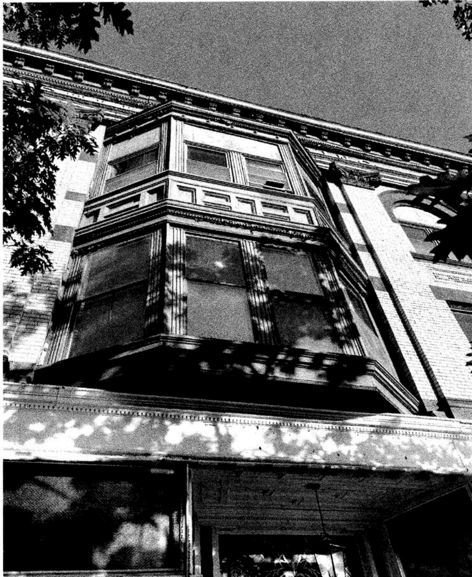
4. Main Street Bay Window – The exterior bay window trim currently painted brown is galvanized metal. This galvanized metal will be scraped of loose paint, primed, and painted brown to match the new Pella “Reserve” historic windows. The perimeter of the bay window where it meets the masonry building will have backer rod and sealant installed at the joint. The windows will be replaced with new Pella Reserve double hung operable windows.
