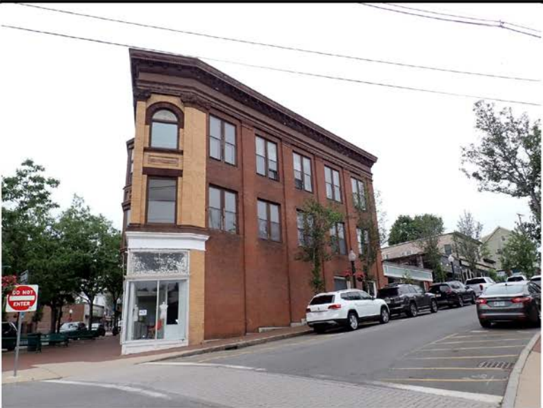
5. North elevation, view south
