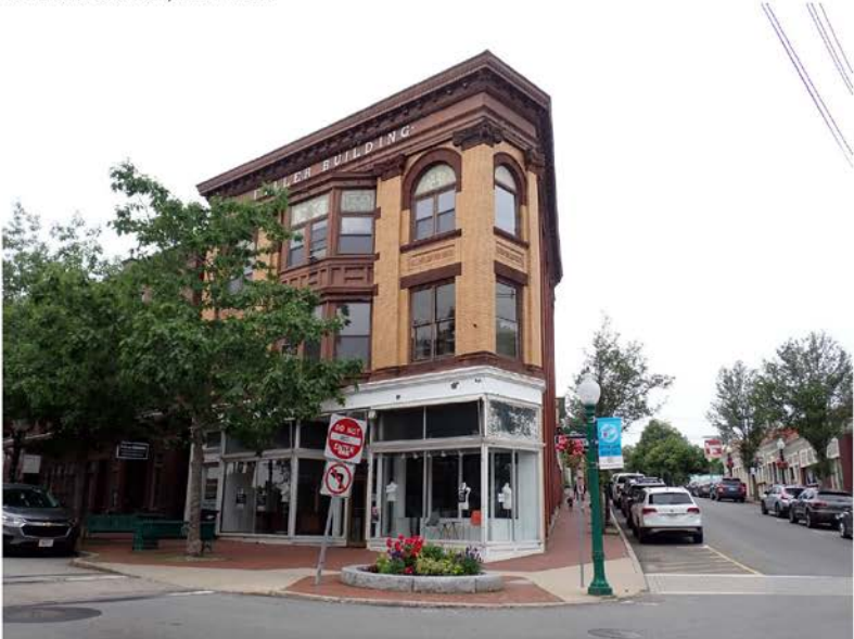
2. East elevation, view southwest
