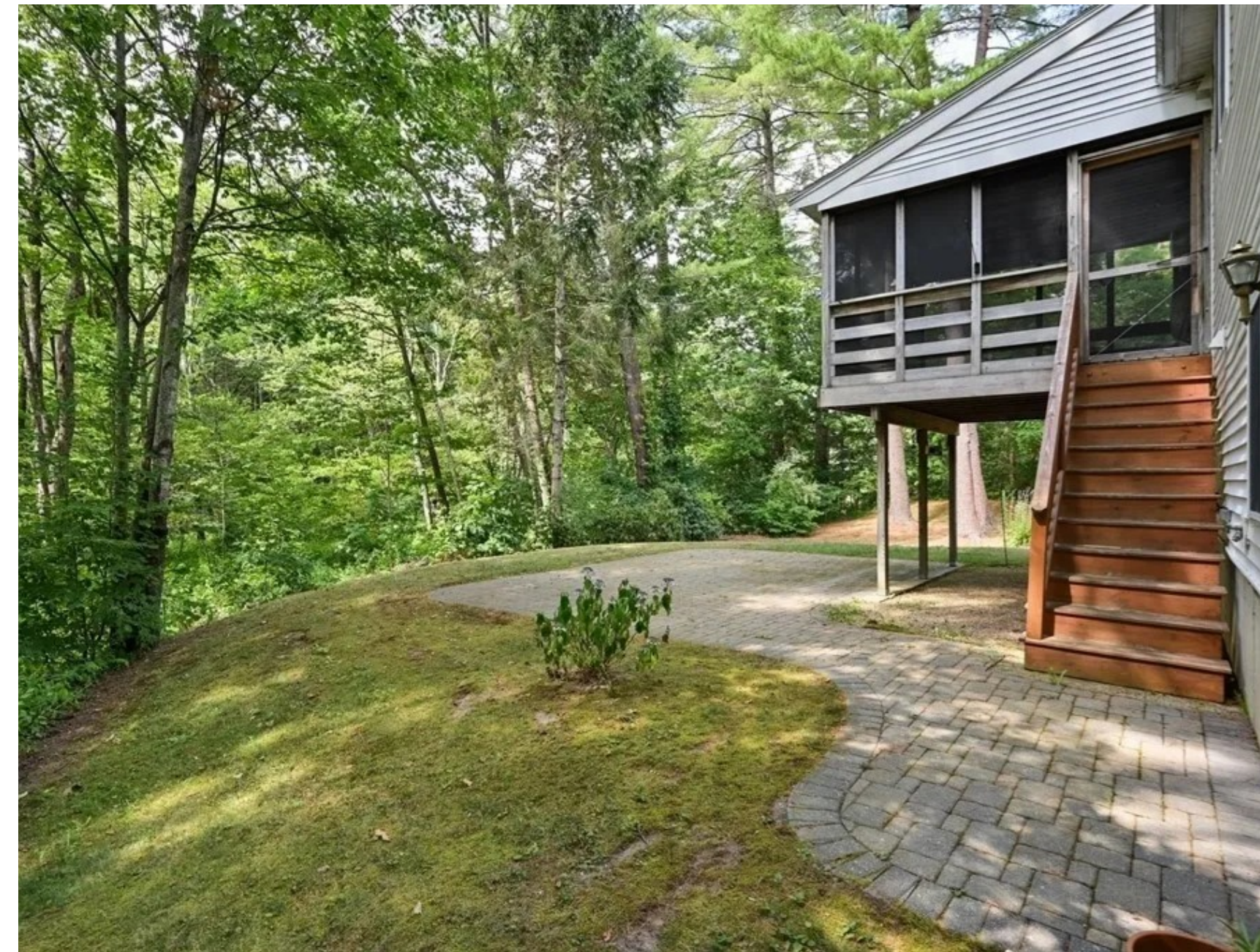
Rear porch expansion area, note patio
