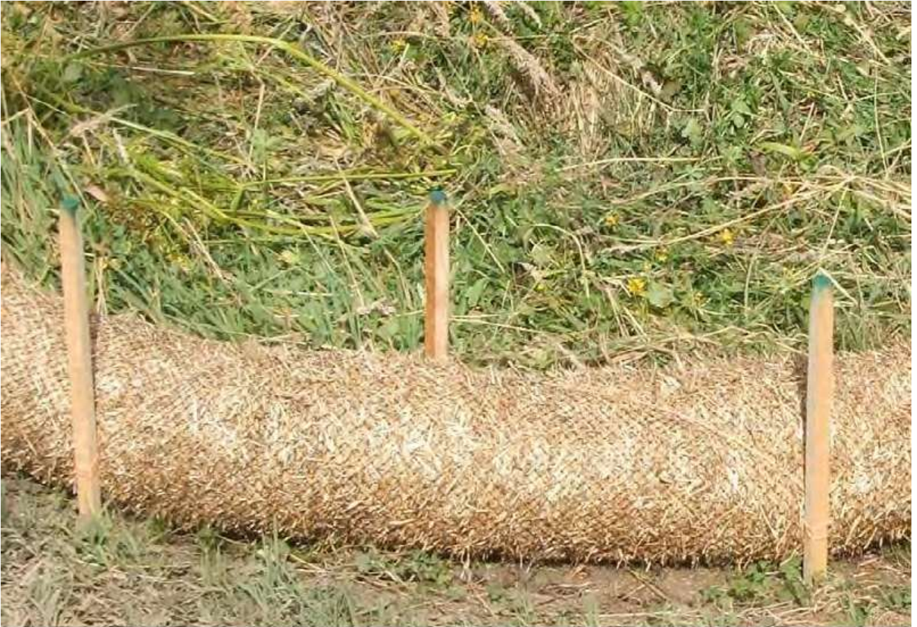
STRAW WATTLE – SHALLOW SLOPE ( \leq 4:1 ) (ALTERNATE STAKING)
