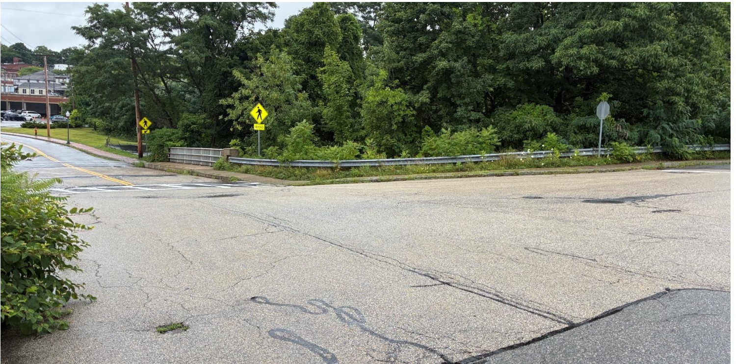
Photo #4: Corner of Chestnut Street and Water Street, facing northwest
