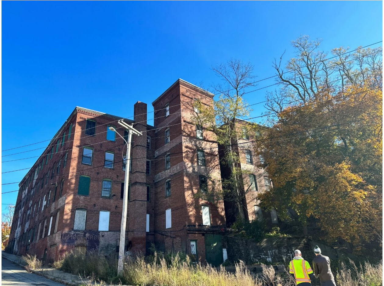
7. Street view of rear of Northern wing from Chestnut Street (Spring 2024)
