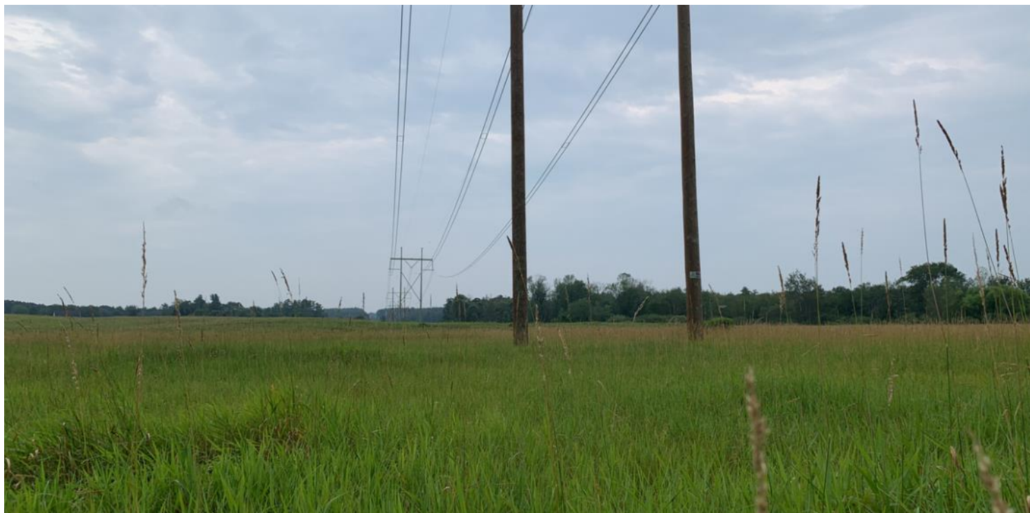
Photo #13: View of wetland AM-W17 and Structure 288 on Line 394.
