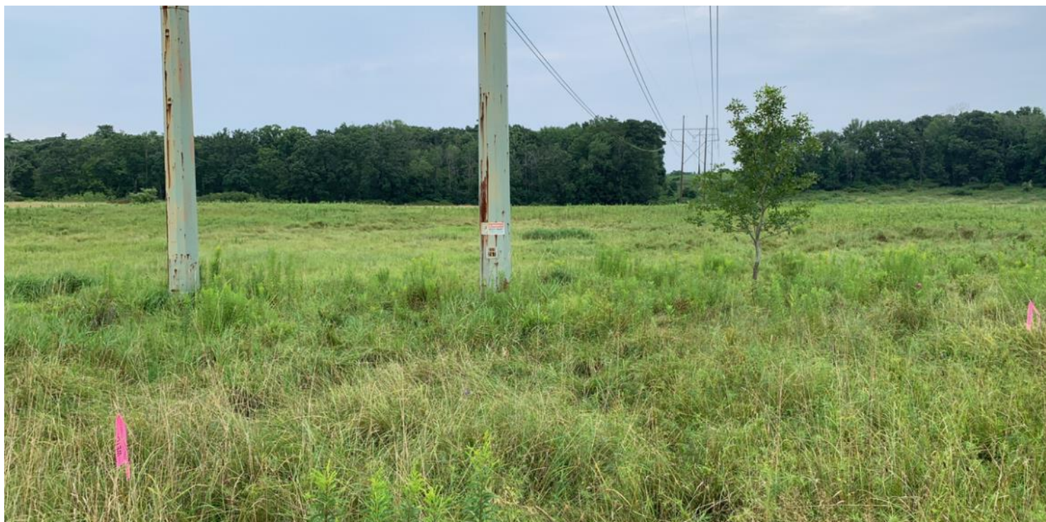
Photo #12: View of wetland AM-W16 and Structure 287 on Line 394.
