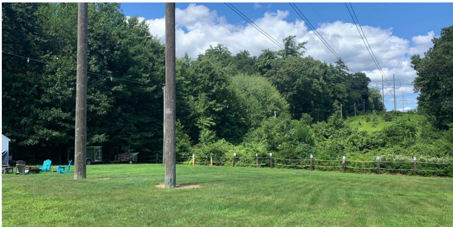
Photo #6: View of Structure 276 on Line 394, with wetland AM-W10 behind the fence.
