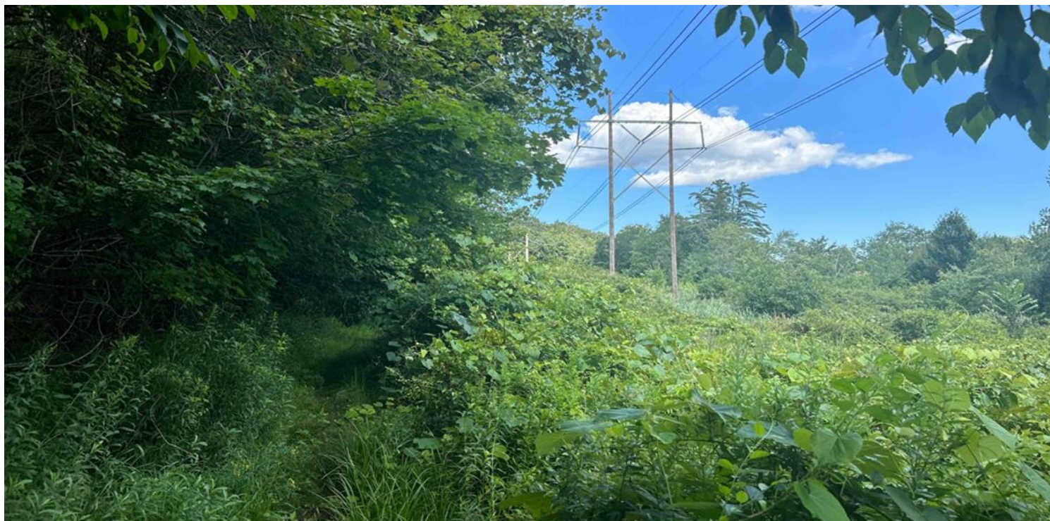
Photo #1: View of Buffer Zone adjacent to wetland AM-W5 between Structures 267 – 268 on Line 394.
