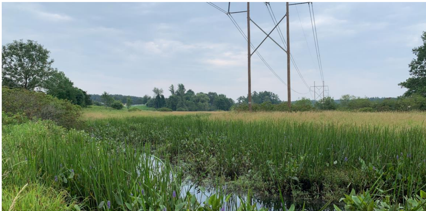
Photo #11: View of stream AM-S15 and Structure 286 on Line 394.
