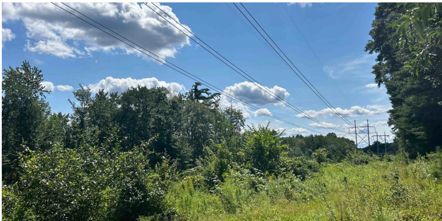
Photo #2: View of Structure 267 on Line 394, in wetland AM-W5.
