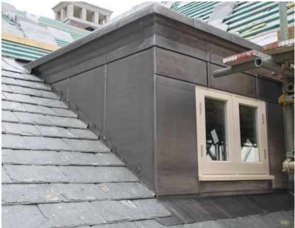
LEAD COATED COPPER DORMER
