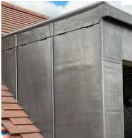
LEAD COATED COPPER DORMER
