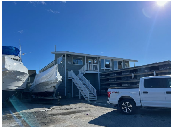
8. View south of existing marina office
