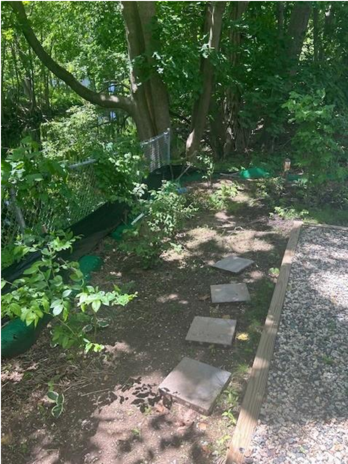
Rear Planting and Stone Infiltration Edge
