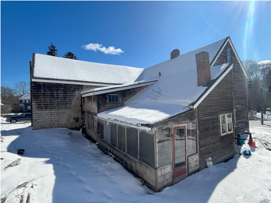
View of the north-facing rear elevation.
