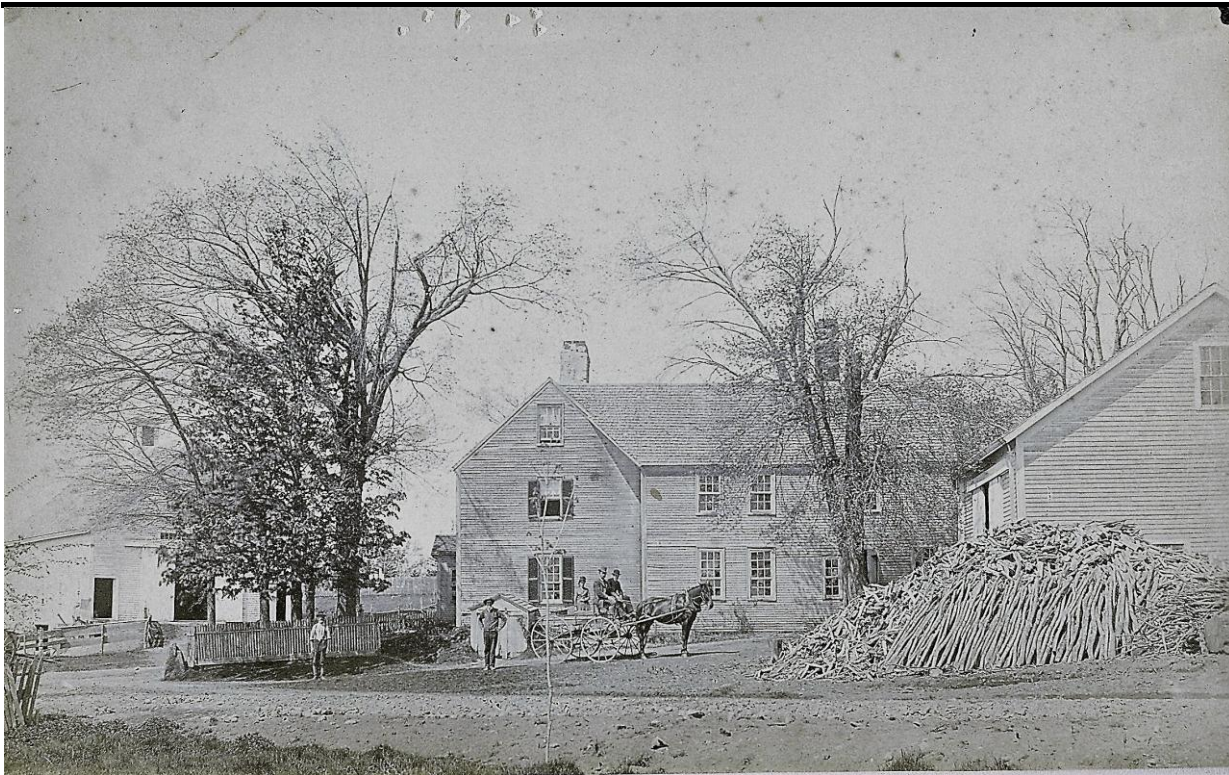
Photograph dated 1893. Note the 9/6 sash and barns in the foreground and background. Source: Amesbury Historical Commission.
