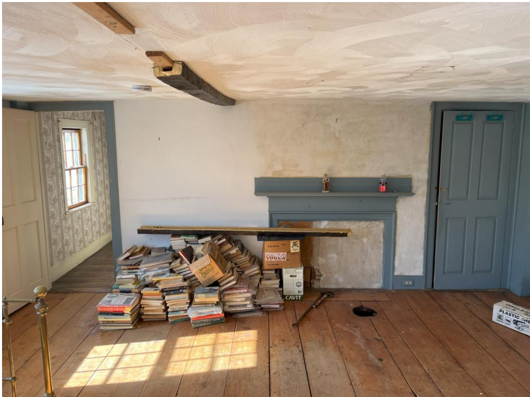
East chamber facing west capturing chimney elevation.
