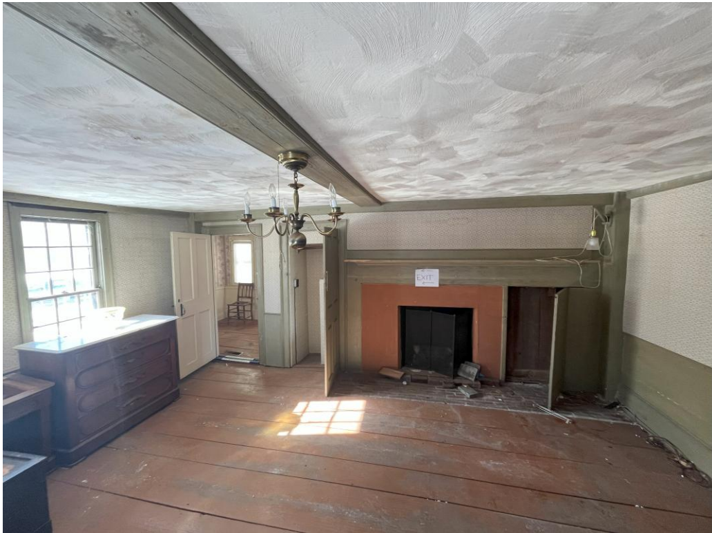
East room facing west. Note the bridging summer, framing at corners, wainscoting, baseboard, architraves, doors and pine floors.
