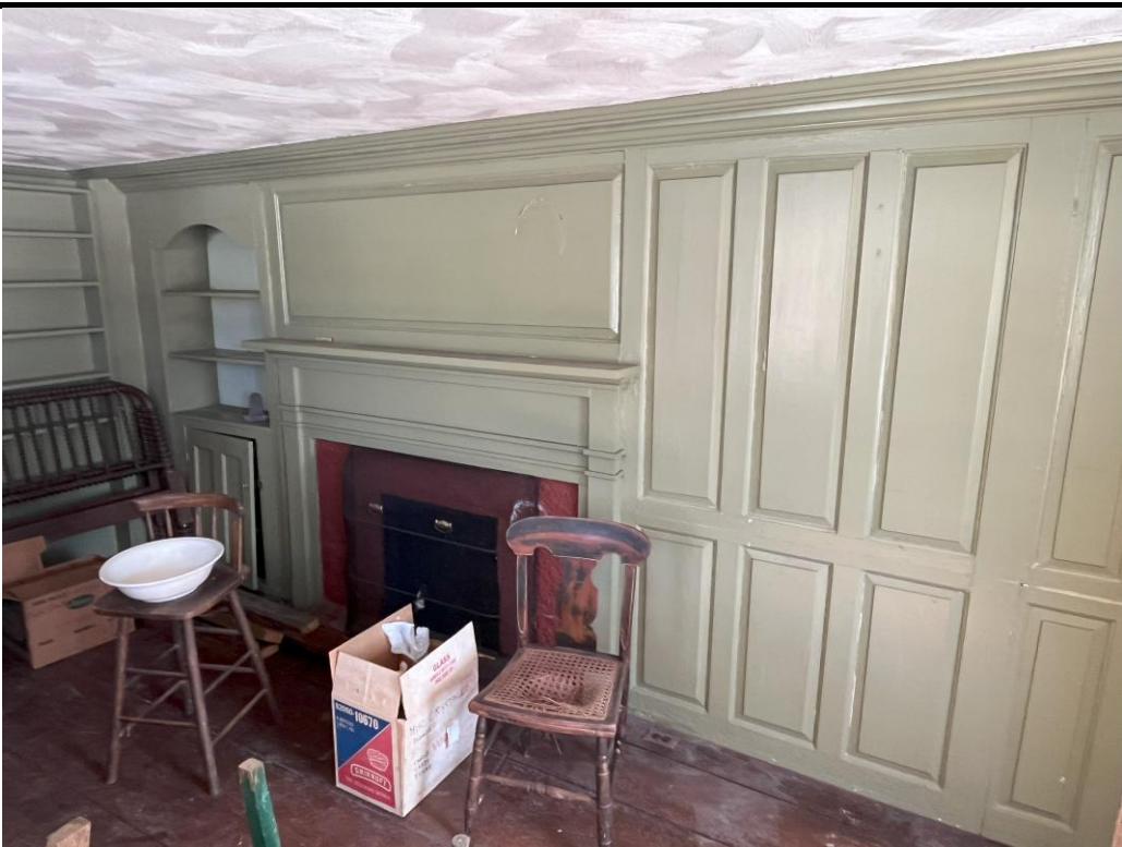
West room chimney wall. Note paneling, cornice and mantel shelf.
