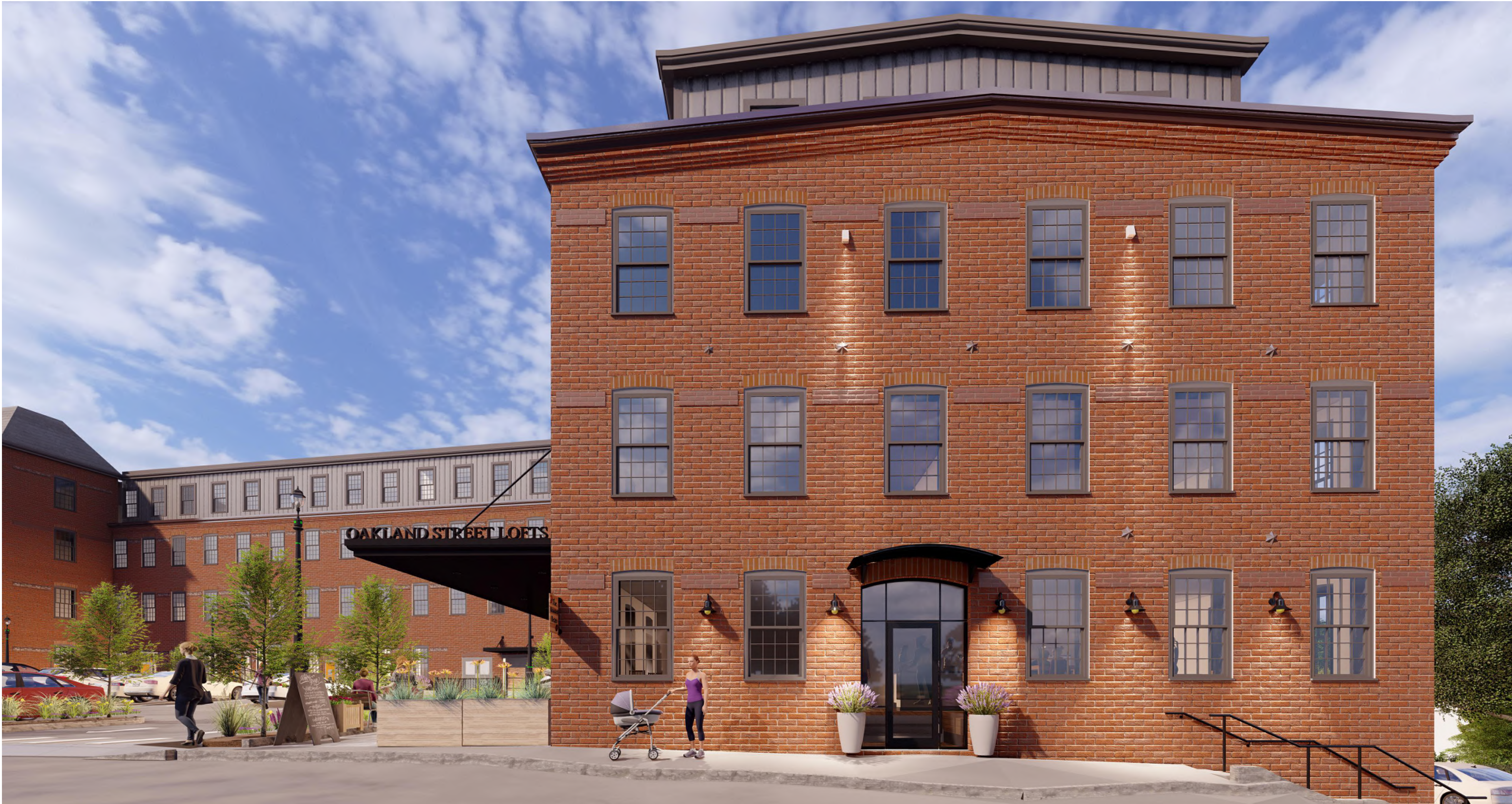
VIEW FROM OAKLAND STREET
