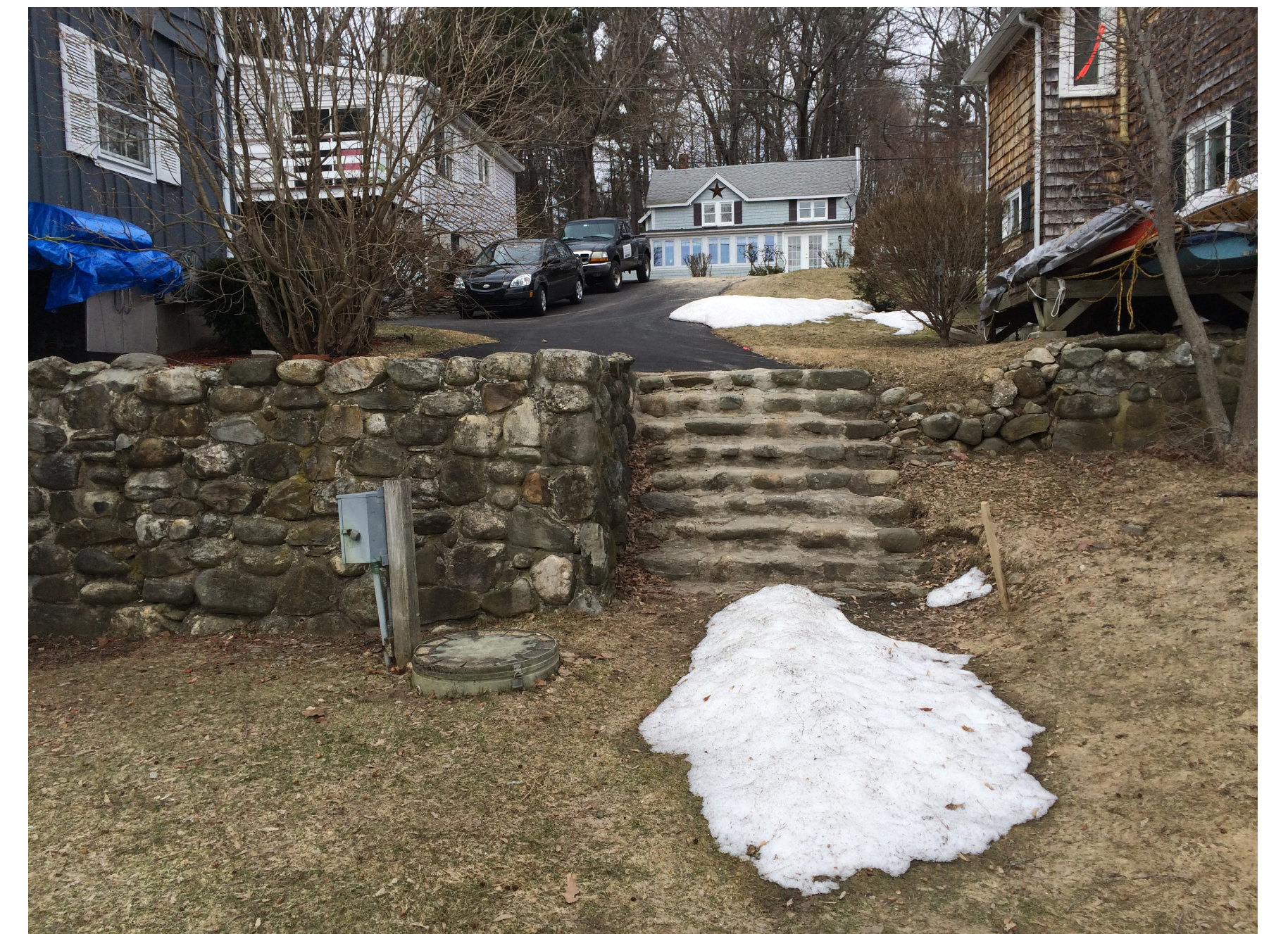
View to east of house towards road
