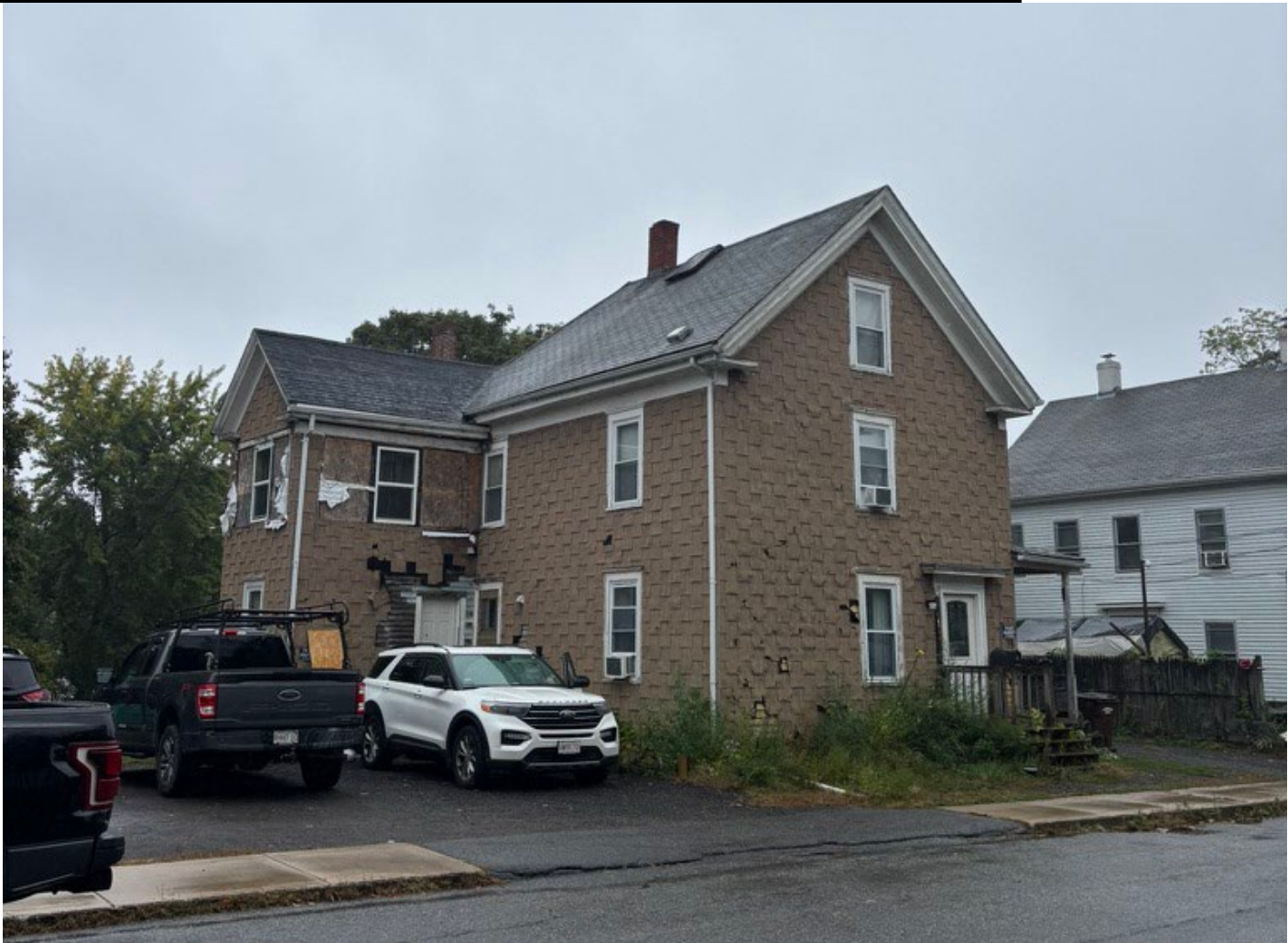
View from Prospect Street, looking east.
