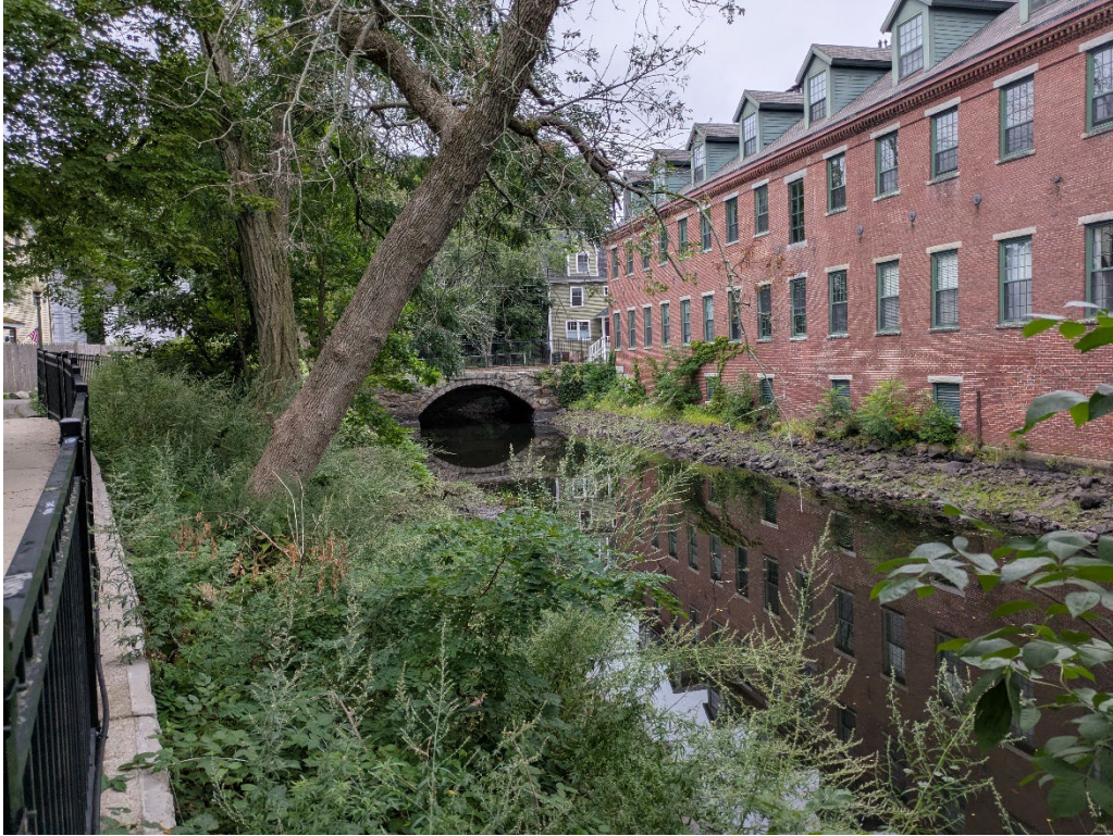
Figure 3 Upstream view of the Pond Street bridge.
