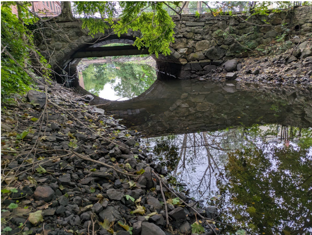
Figure 4 Downstream view of the Pond Street bridge.
