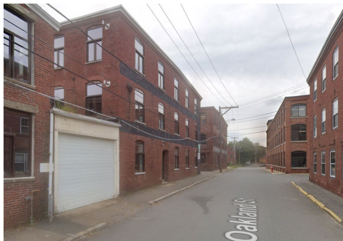
View of buildings south of site on Oakland Street
