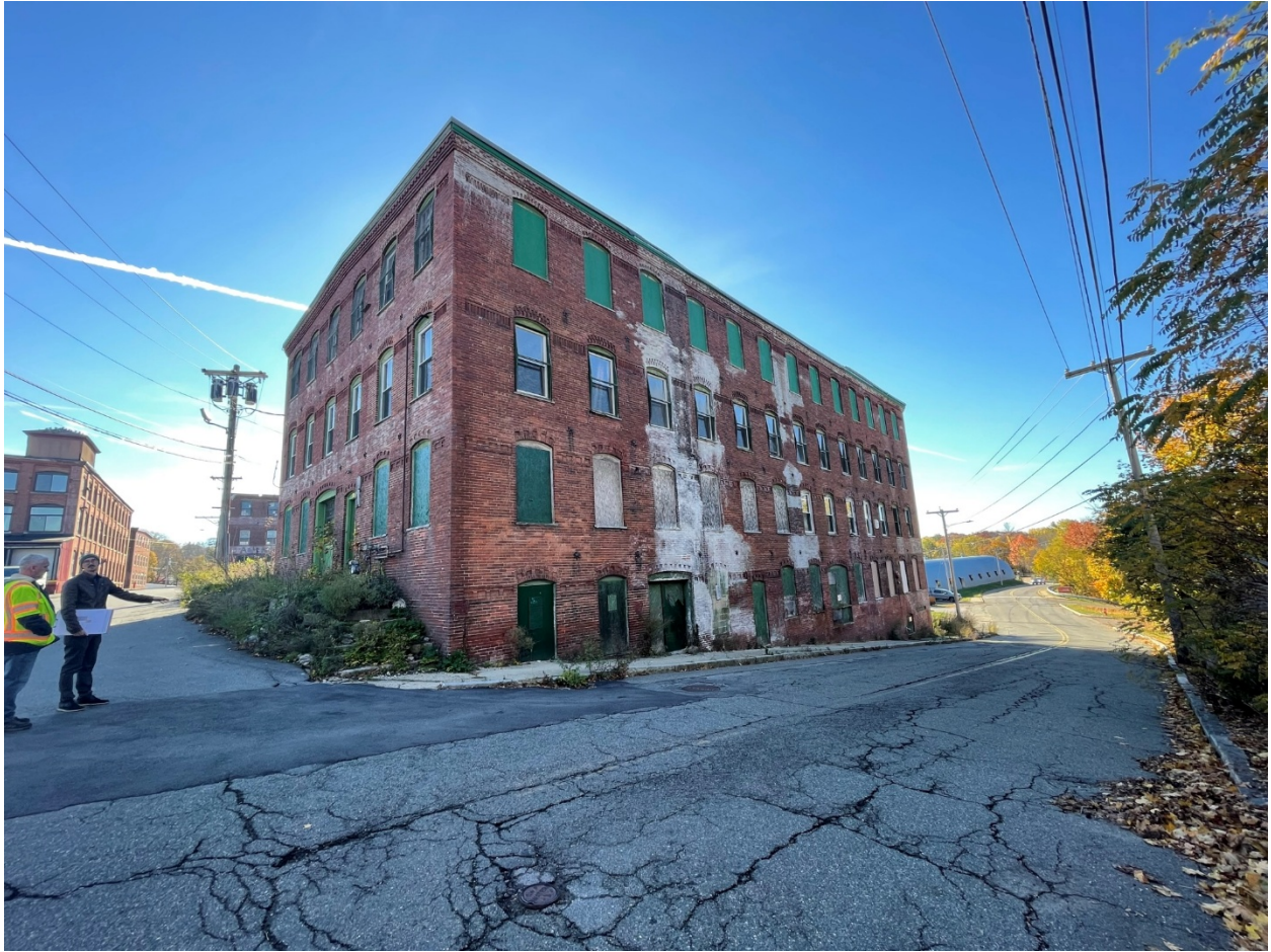
6. Street view of Northern wing from Oakland Street & Chestnut Street (Spring 2024)
