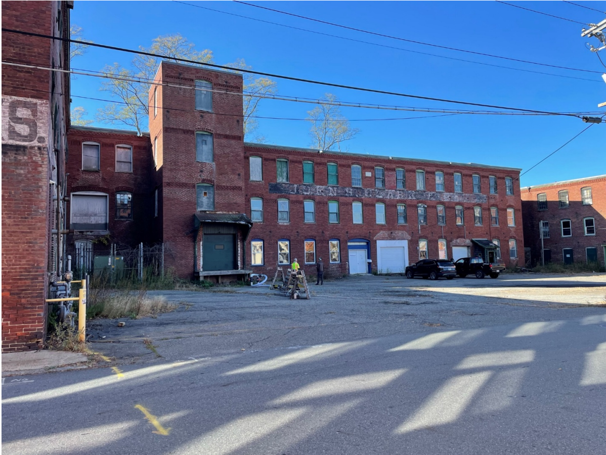
4. Street view of middle wing from Oakland Street (Spring 2024)
