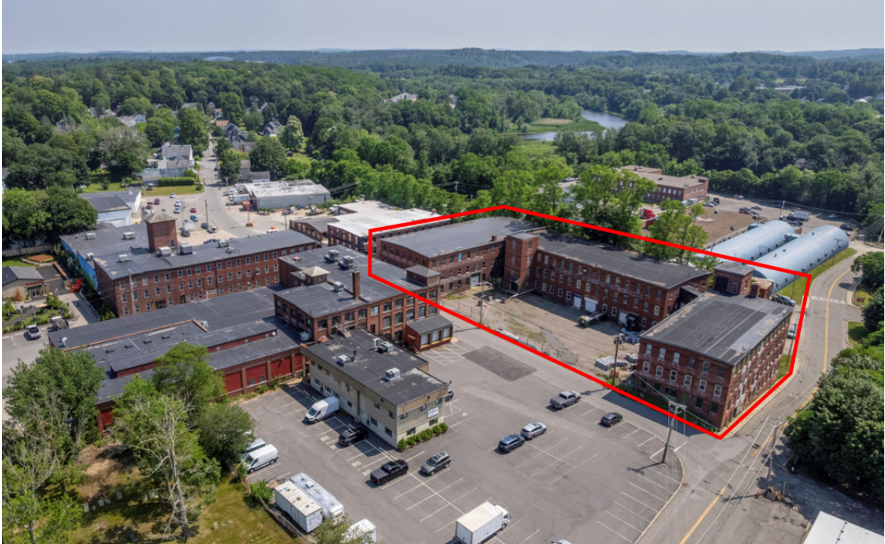
1. Aerial view from Chestnut Street (Summer 2025)
