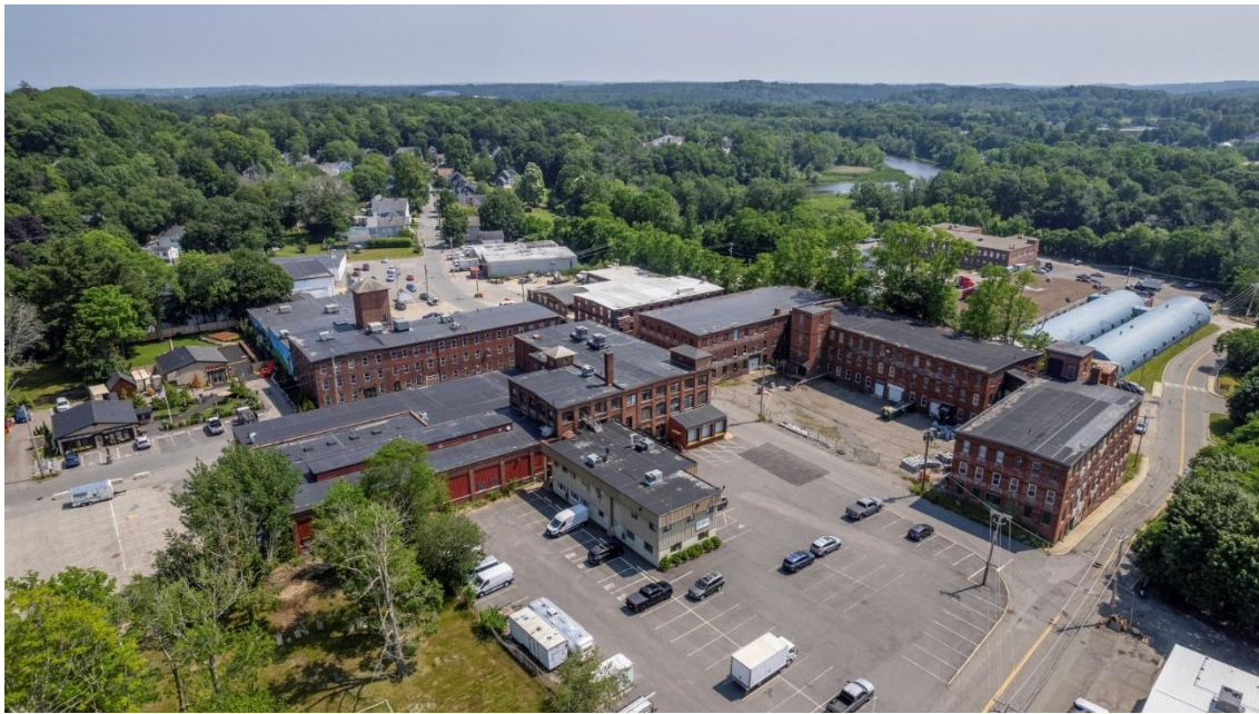
View of site looking down Chestnut Street (right side)
