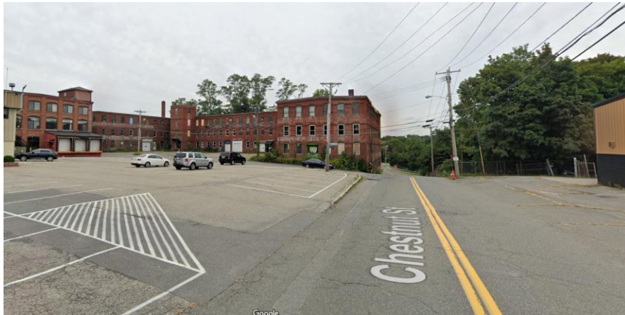
View of buildings east of site on Chestnut Street
