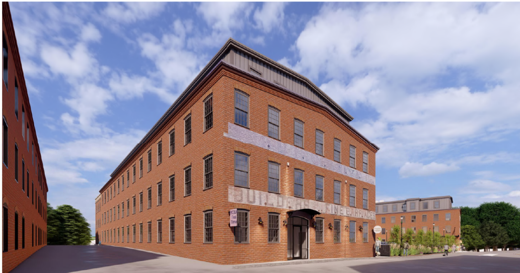
VIEW FROM OAKLAND STREET
