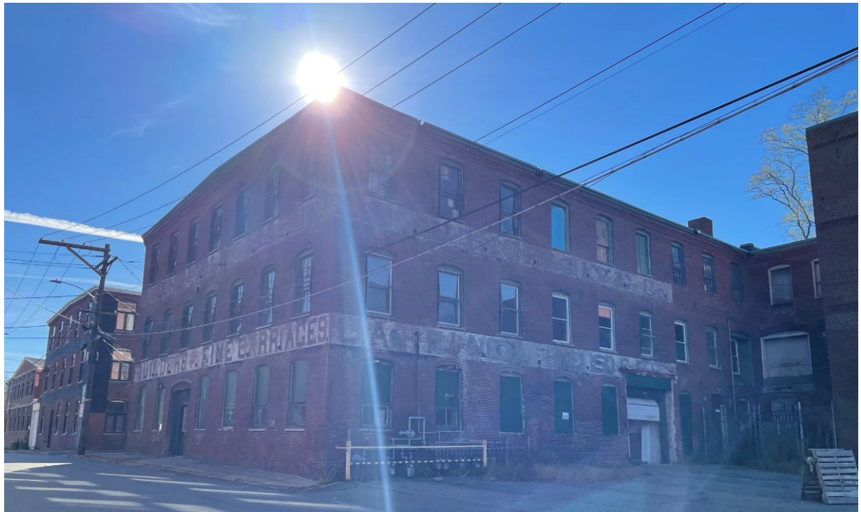
3. Street view of Southern wing from Oakland Street (Spring 2024)
