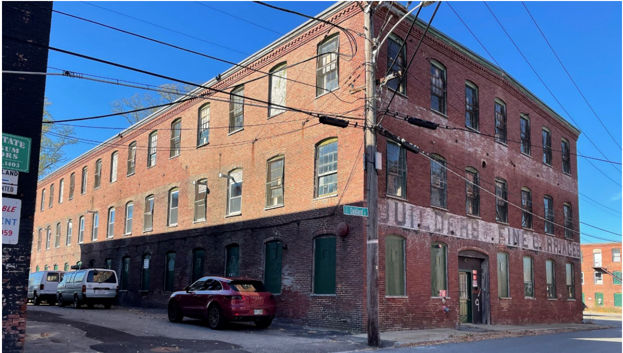
2. Street view of Southern wing from Oakland Street (Spring 2024)
