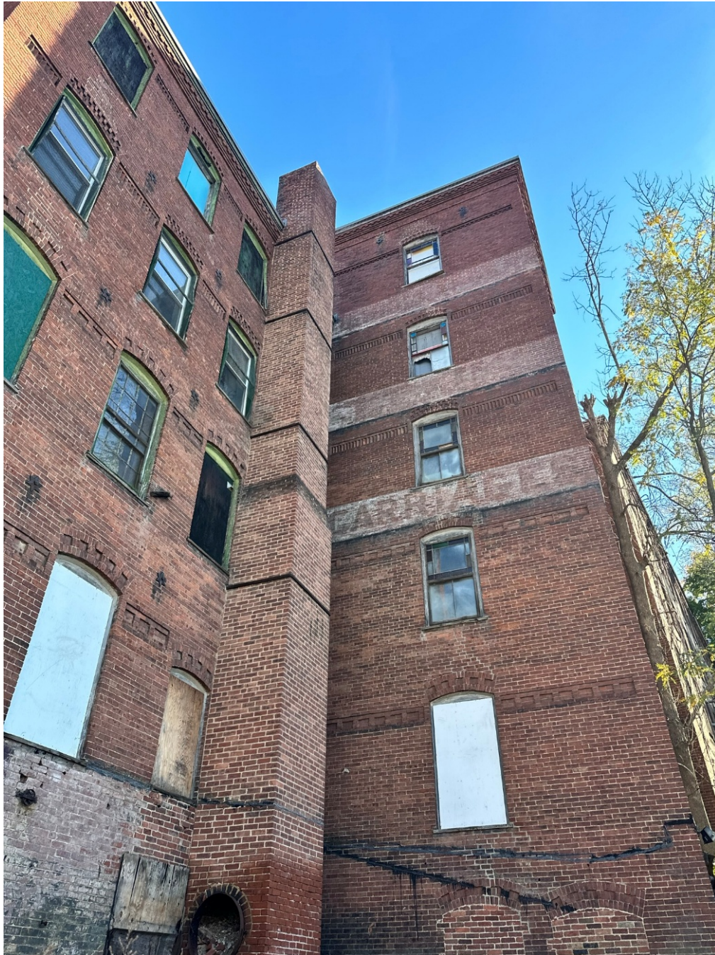
8. View of tower & chimney at base of hill (Spring 2024)
