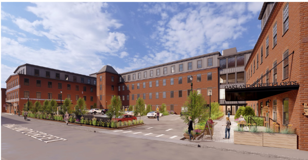
VIEW FROM OAKLAND STREET
