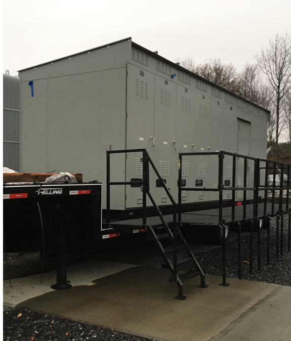
Mobile Switchgear
