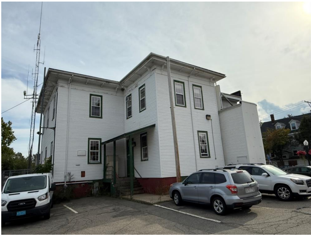
Looking southwest at 1884 addition
