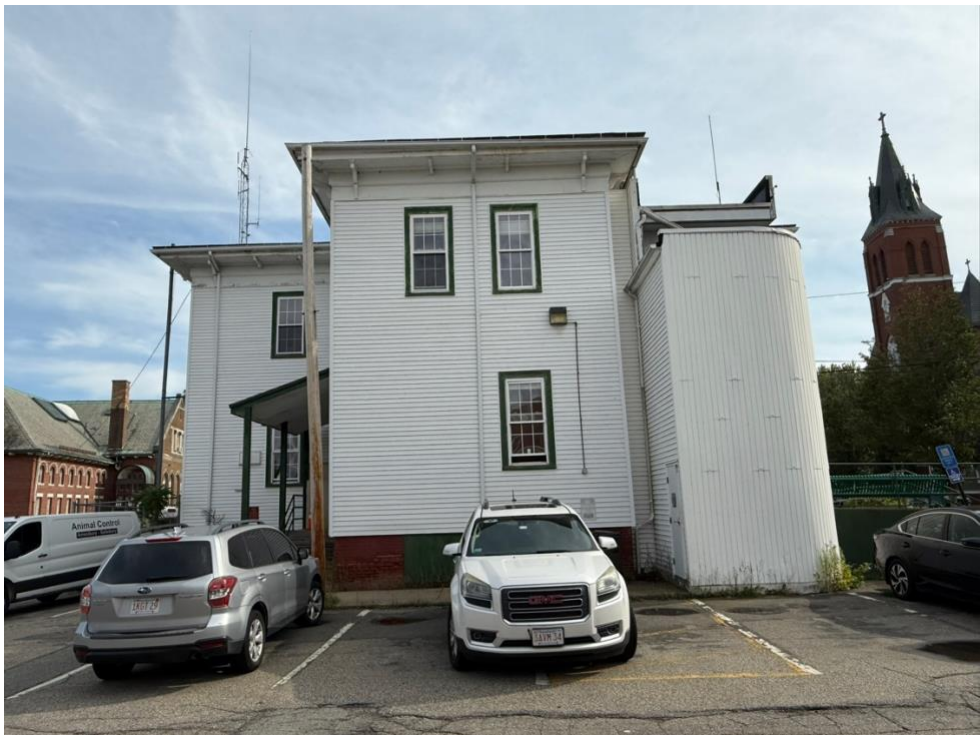
North elevation – 1884 addition at center and 1981 addition at right
