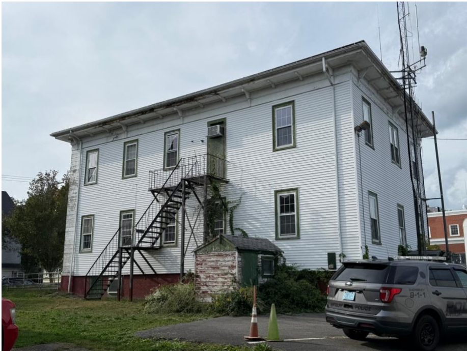
South and east (rear) elevations
