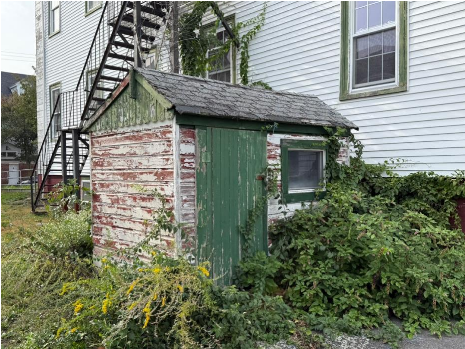
Shed at southeast corner
