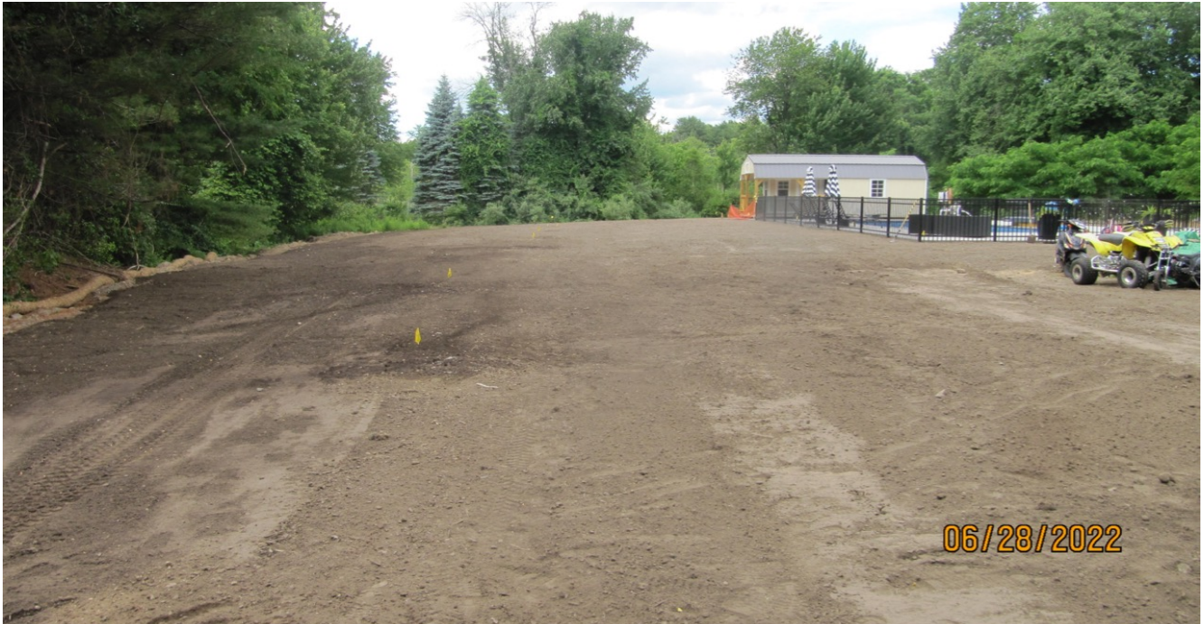
Photo C. Property loamed and sprinkler system being laid out.
