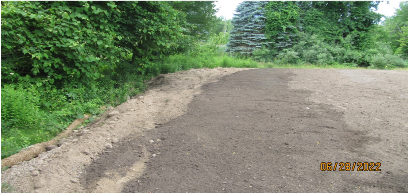
Photo E. Edge of filled area after loaming. Edge needs regrading and stabilization before coir logs can be removed.
