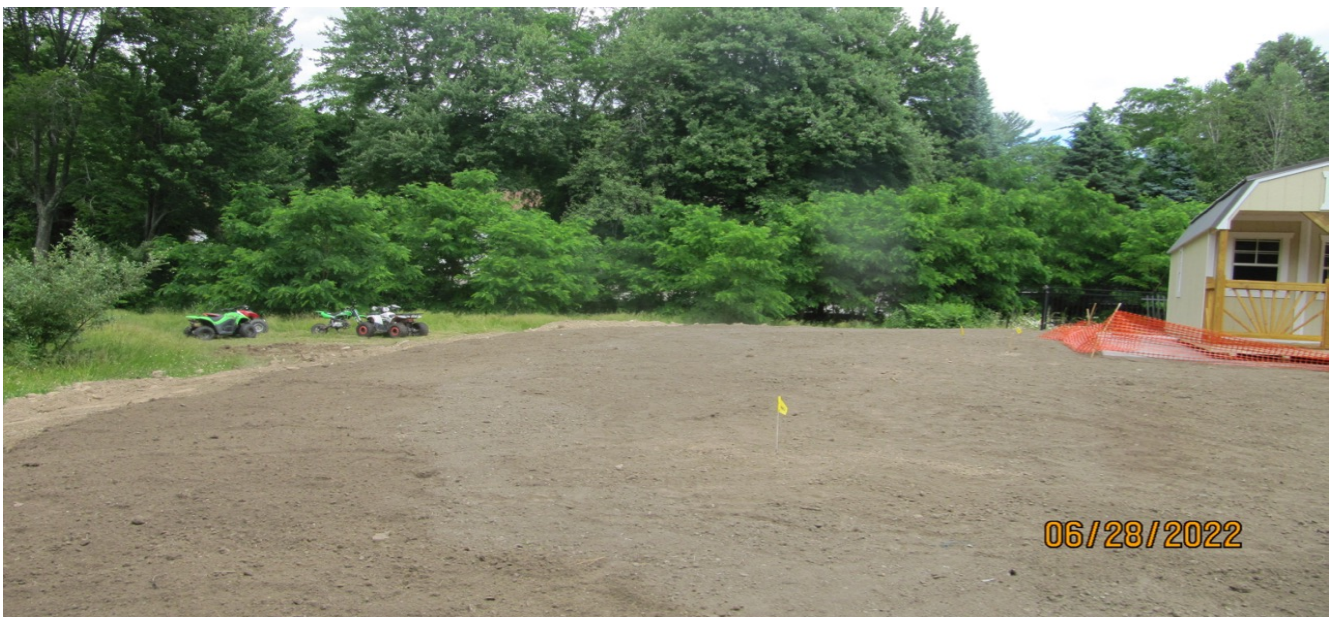
Photo F. Property loamed and sprinkler system being laid out.
