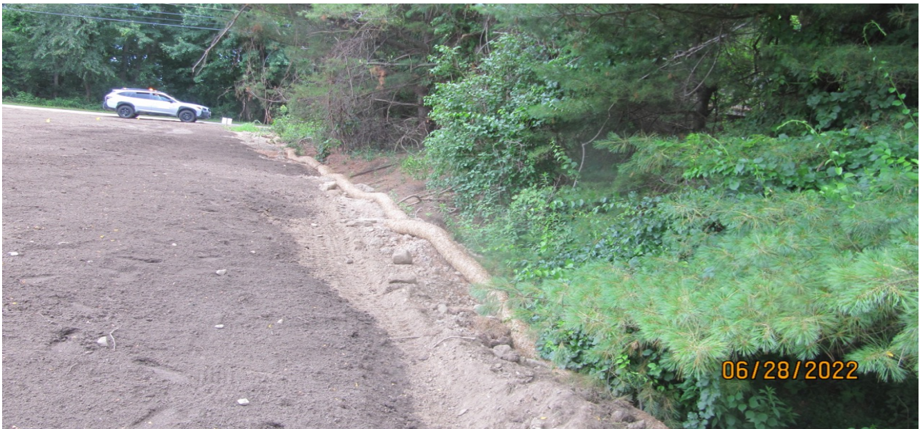
Photo D. Coir logs installed around perimeter of regraded filled area. Coir logs should be staked in place.
