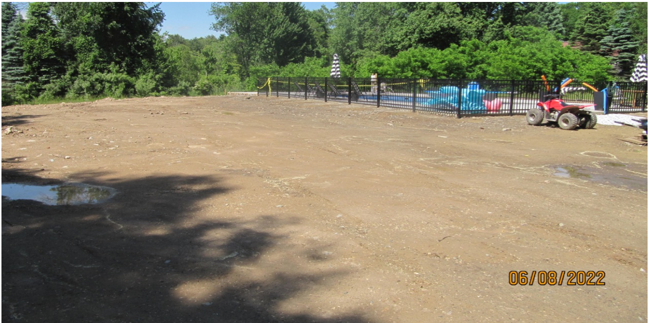
Photo B. Southwestern end of property after being filled with sand and gravel and then regraded,
