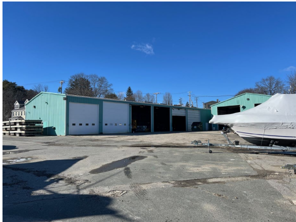
7. View N of existing buildings and parking
