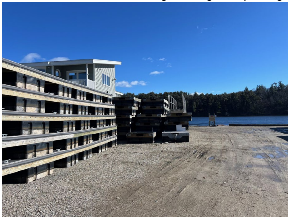
9. View south at west end of site
