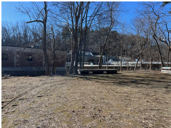
10. View west toward treatment plant
