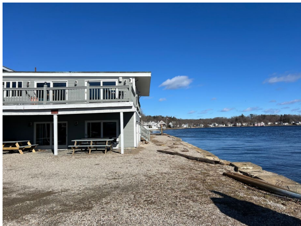
1. View NE along Merrimack River
