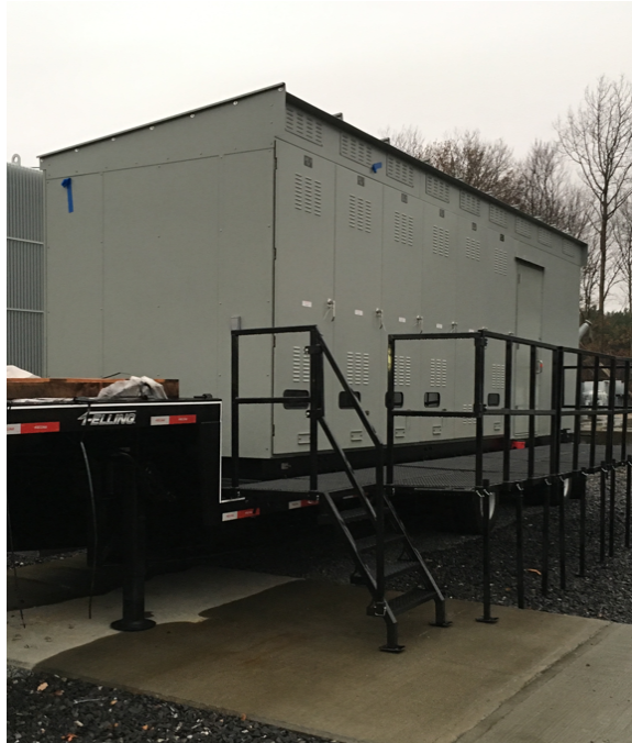
Mobile Switchgear
