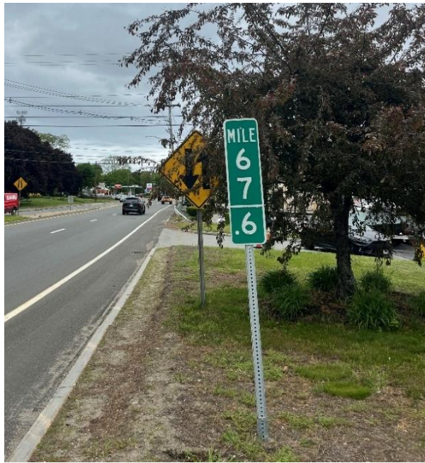
Figure 15: Vegetation blocking lane median drop
