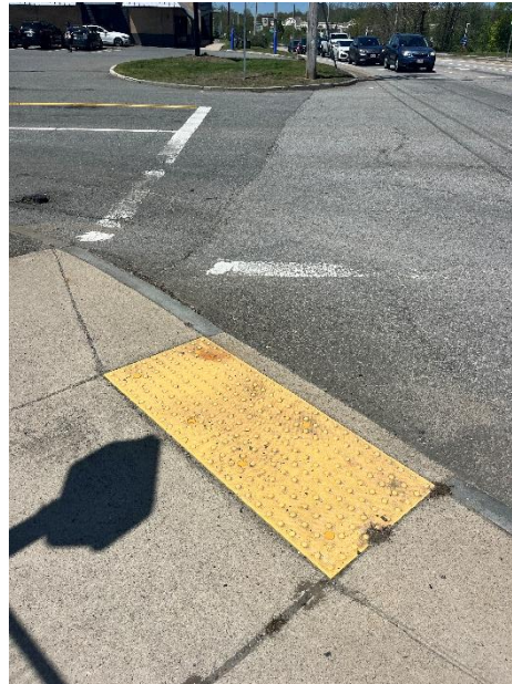
Figure 10: Pedestrian ramp on southeast corner
