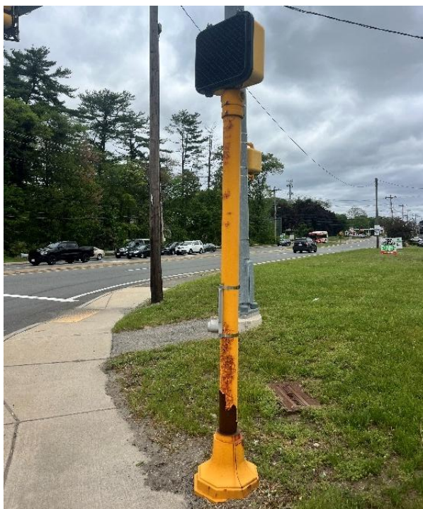
Figure 18: Non-APS pushbuttons on southeast corner
