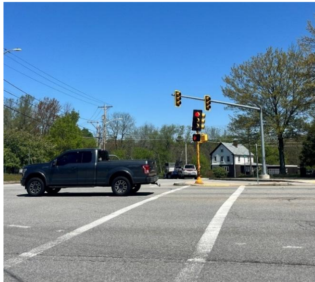
Figure 7: Crooked signal head on slip lane median island
