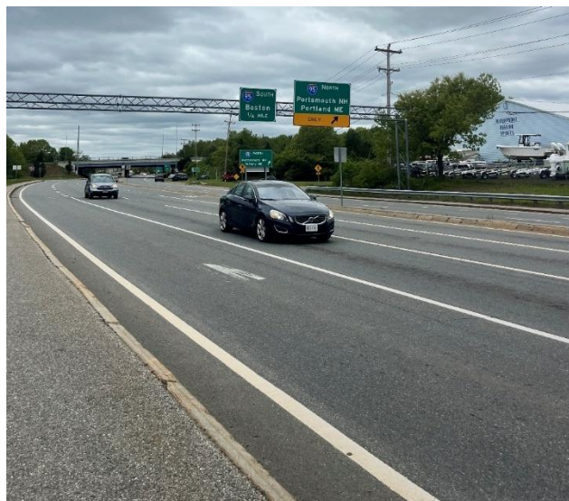
Figure 14: Missing pavement markings for designated right turn only lane for the eastbound approach to the intersection.
