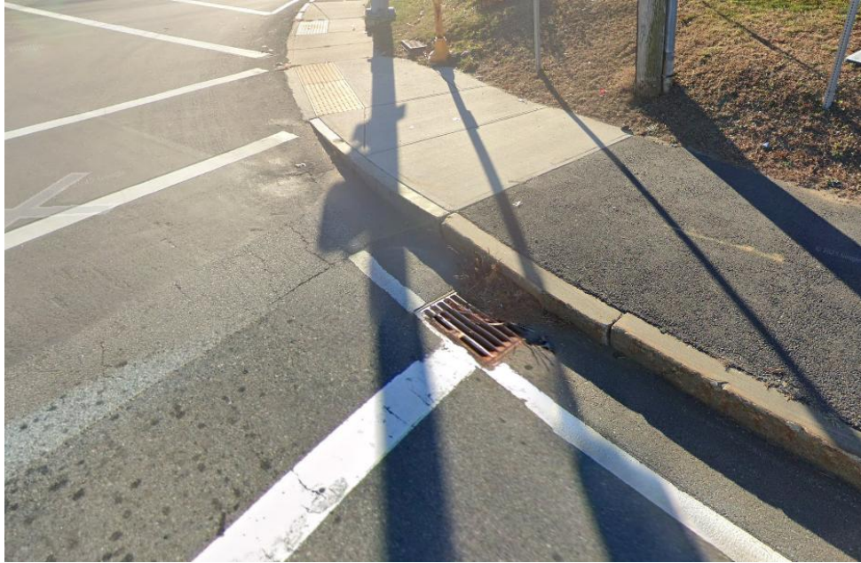
Figure 20: Parallel catch basin grate on southwest corner
