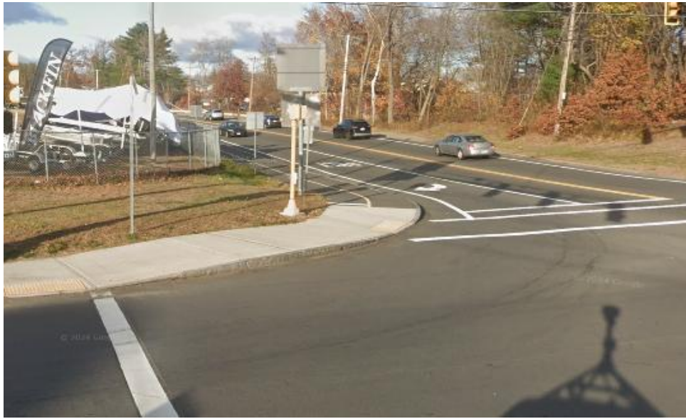
Figure 12: View of large turning radius on northwest corner
