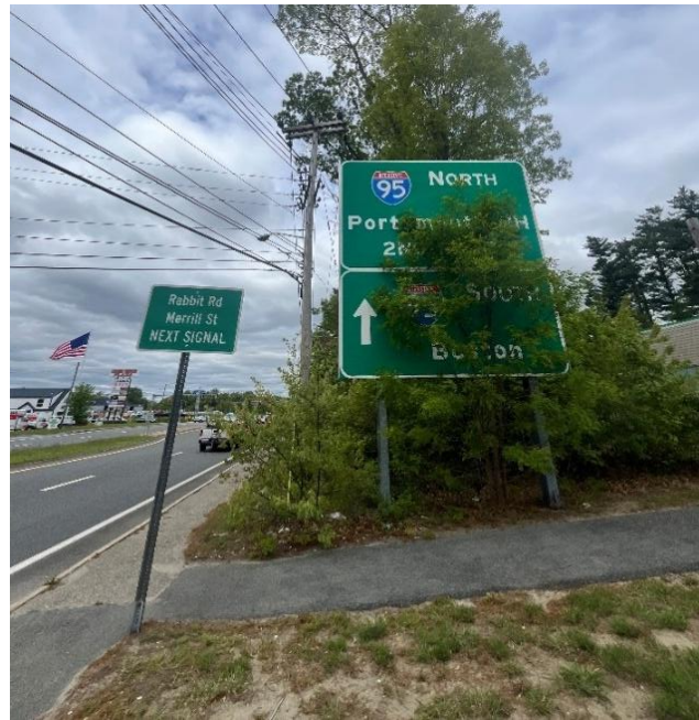
Figure 16: Vegetation in front of I-95 sign westbound
