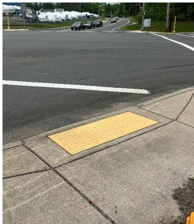
Figure 19: Curb ramps on southeast corner
